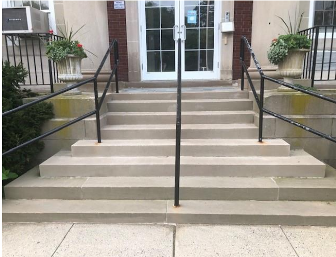
Existing entry steps at front of school
