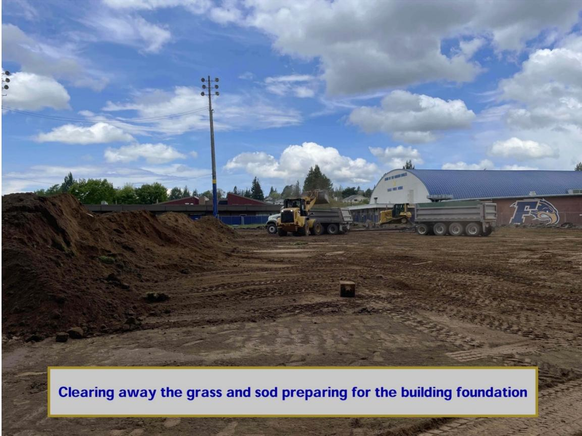
**Clearing away the grass and sod preparing for the building foundation**
