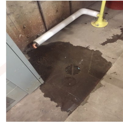
The new eyewash installed is missing signage and weekly checklist. The drain was blocked and needed to be cleared - corrected
