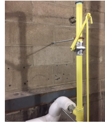
The new eyewash installed is missing signage and weekly checklist. The drain was blocked and needed to be cleared - corrected
