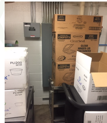
Blocked electrical panels - corrected
