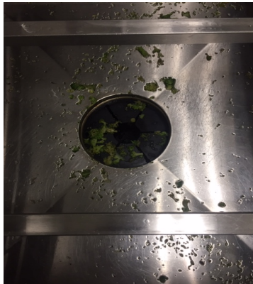
Garbage disposal guards missing- corrected
