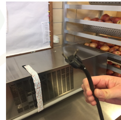
Kitchen fan missing ground prong and damaged prongs - corrected
