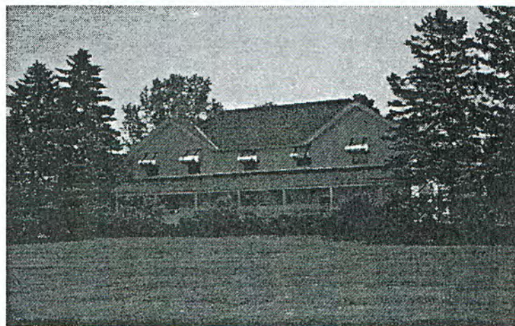
Former Retirement Home and Mrs. Allis' Boarding House Photo by : Shawna Wearne
