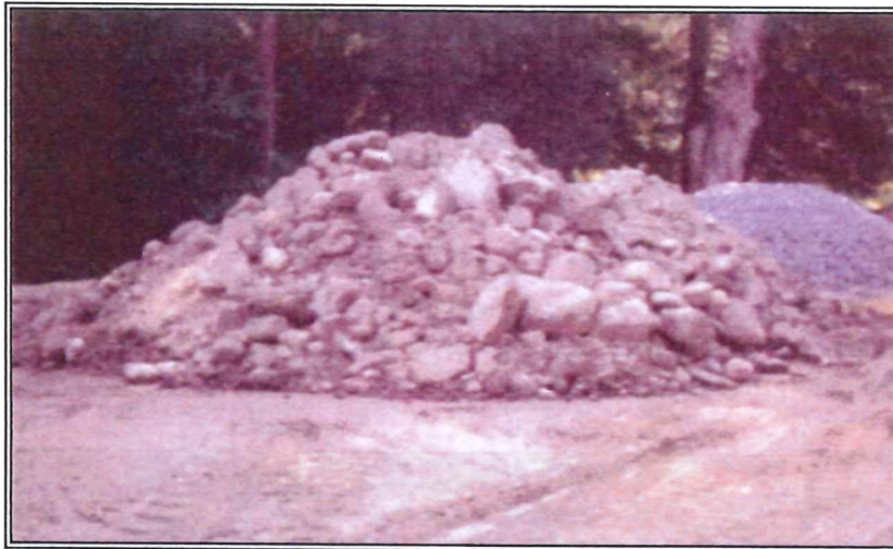
Figure 9. Streambed materials stockpiled for installation within sunken culverts.
