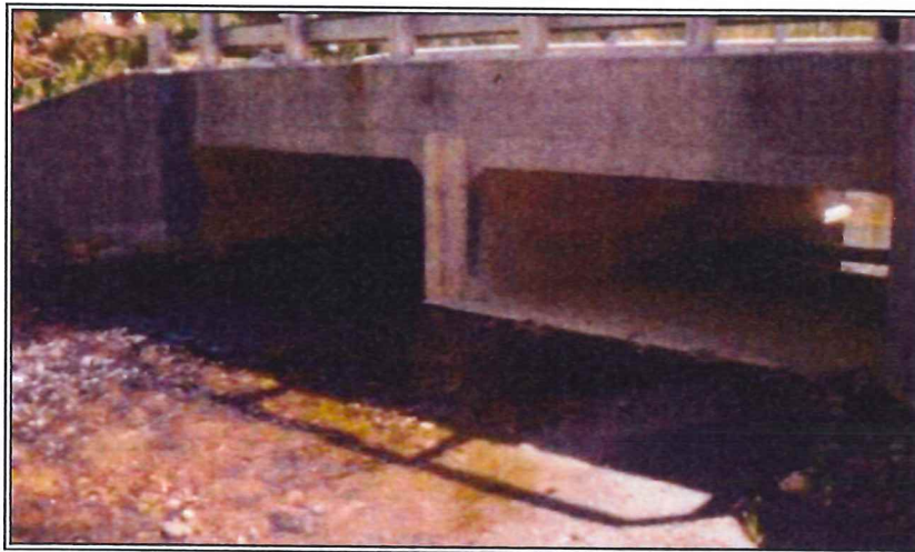
Figure 7. Culvert on left is sunken 1 foot below grade. Culvert at right, installed “at grade” accommodates high stream flows.
