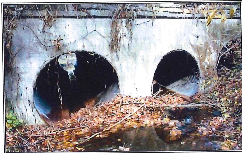
Figure 5. Debris blockage at culvert inlets that blocks fish passage.
