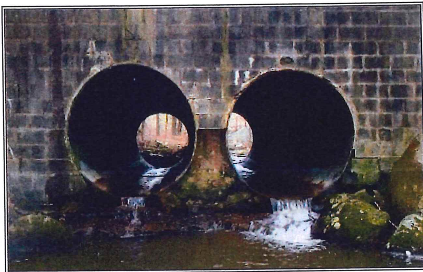
Figure 2. Example of culverts perched above streambed.
