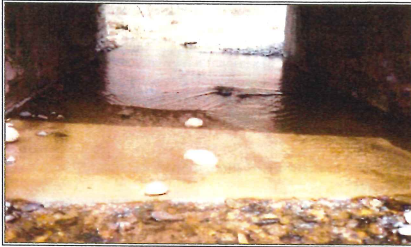
Figure 3. Example of shallow water conditions in a concrete box culvert.
