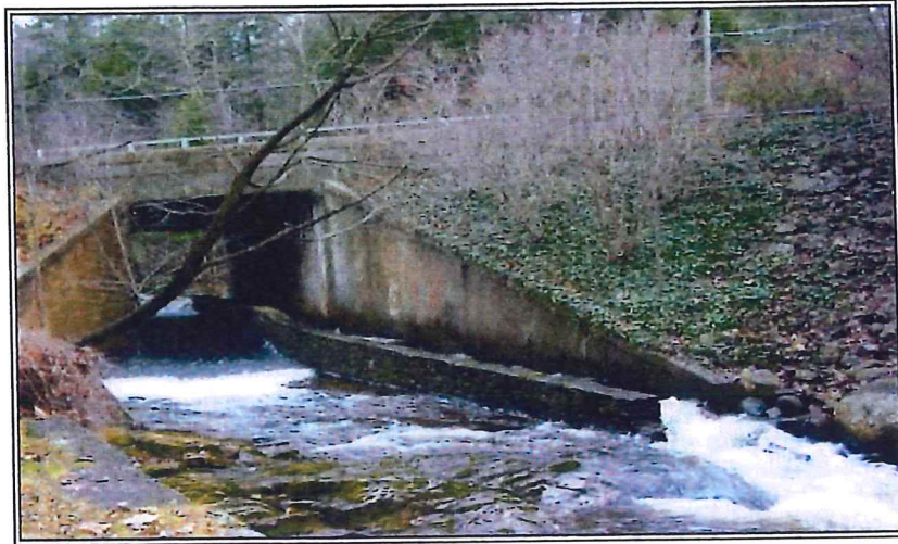
Figure 13. Example of fishway installed within a culvert.
