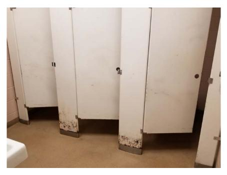
Before construction – noncompliant ADA fixtures and layout, peeling flooring, corroded stalls
