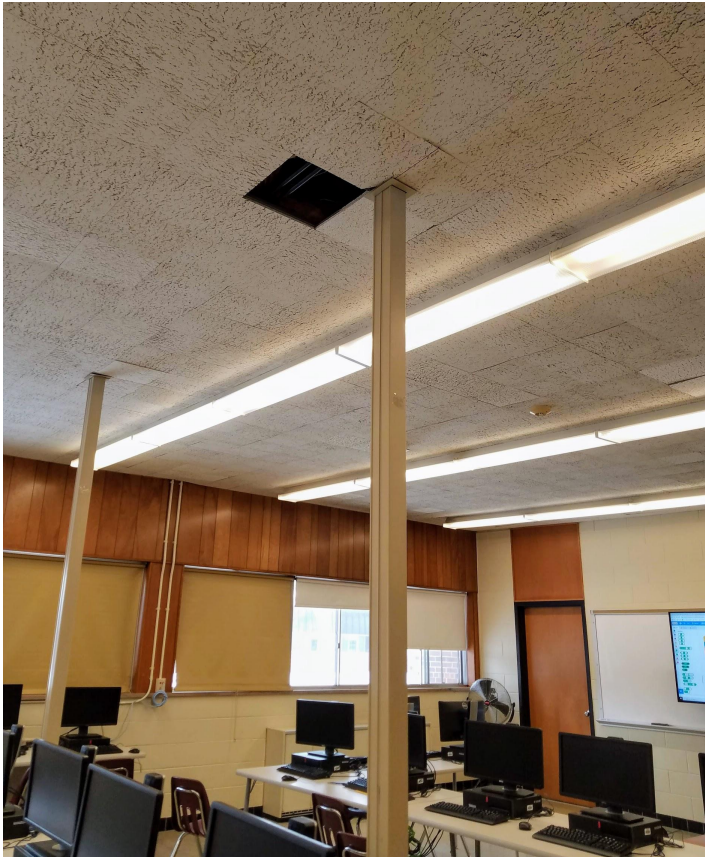
Fluorescent Lights and Poorly Insulated Ceiling Enclosure
