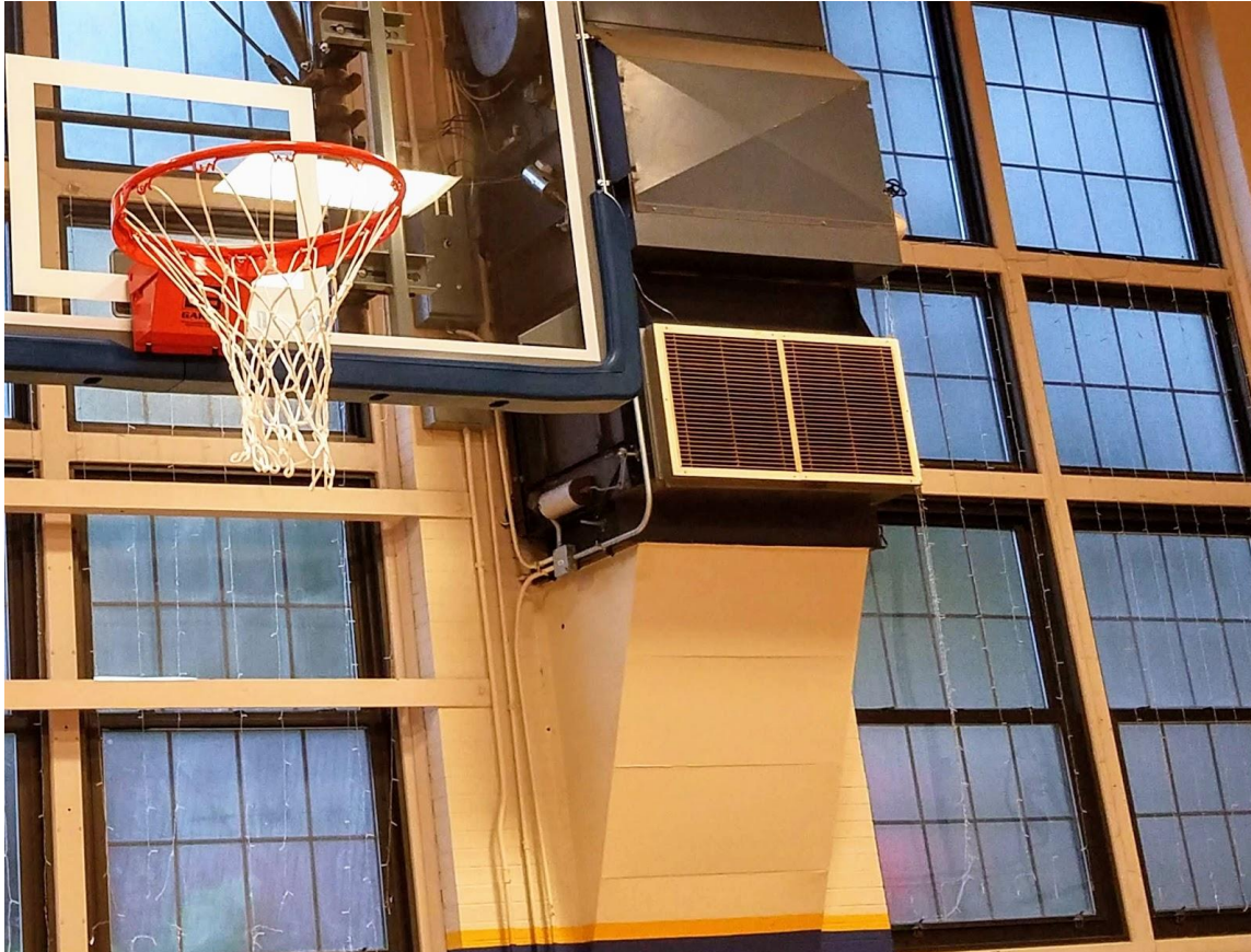
1960's Vintage Air Handling Unit and Poorly Insulated Windows
