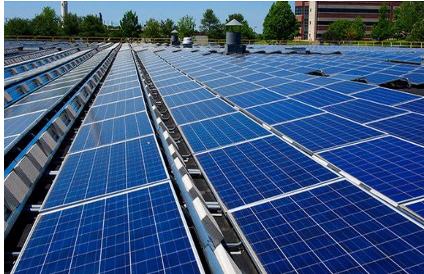
100 kw PV (Photovoltaic) Array
