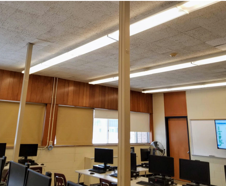
Fluorescent Lights and Poorly Insulated Ceiling Enclosure
