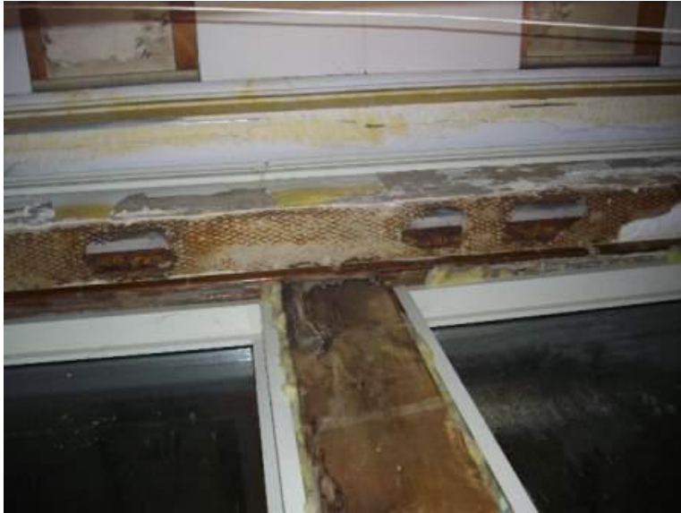
Typical level 3 window head above ceiling.
