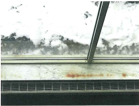
Picture #5: Staining of finish material due to water penetration of slope glazing in "Atrium". Further examples of issues with the "Atrium" are shown further in this photo survey.
