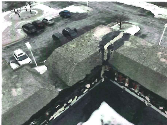
Picture #19: Typical issue for the top of the wall where there is stone coping. Improper prior attempt to fix the coping grout between stones. Roof membrane should go up the wall and under the stone coping.
