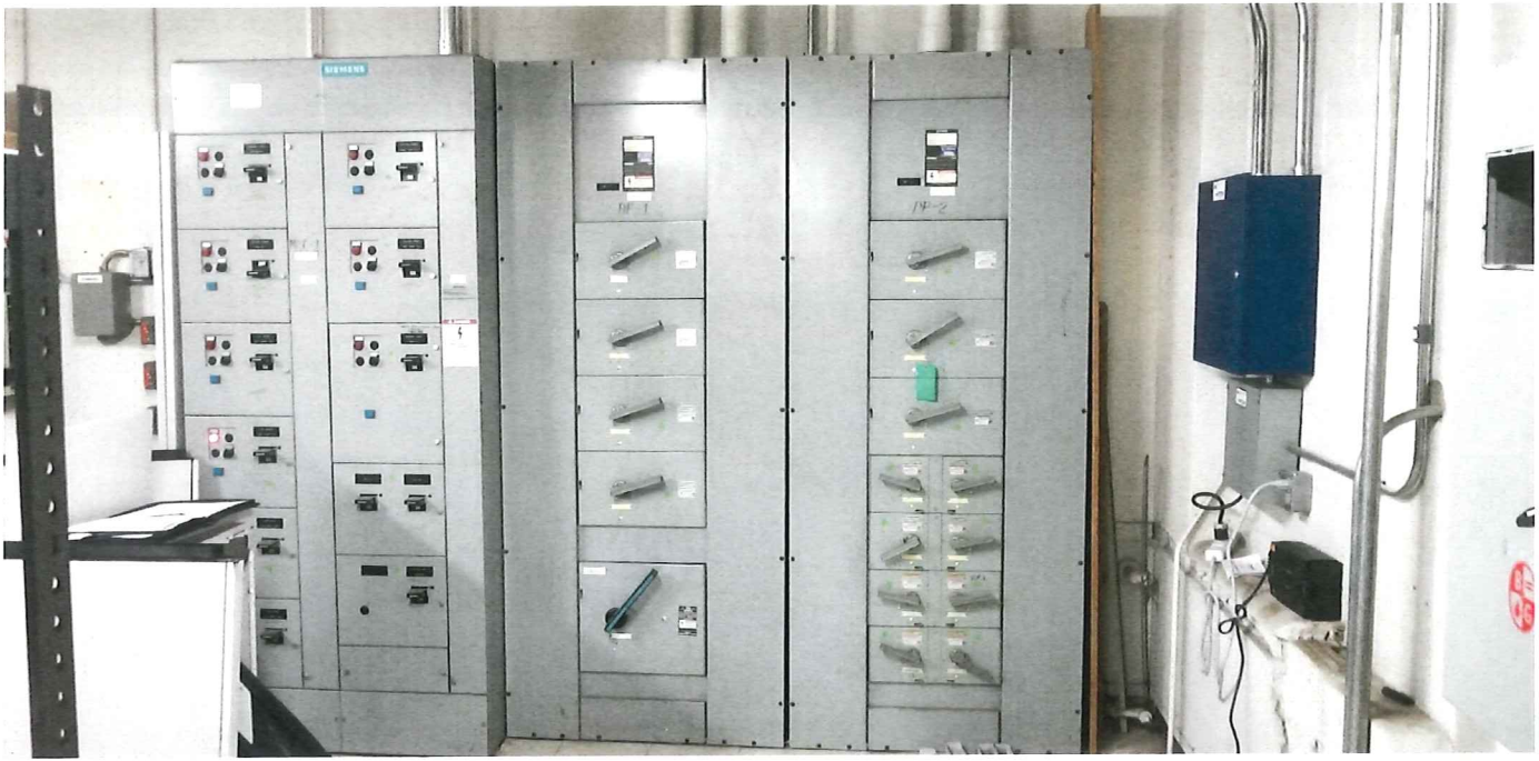
E5 – Distribution Switchboards / Motor Control Center
