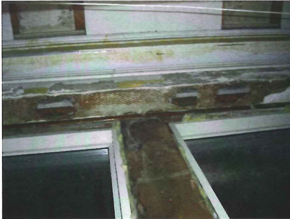
Pictures #42 & 43 (#52 & 53 Similar): Typical Level 3 window head above ceiling.
