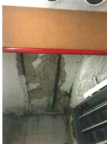
Picture #8: Room under exterior walkway. This room has no area above it or grade. Damage is caused by the infiltration of water and environmental containments. Rooms should be demolished.
