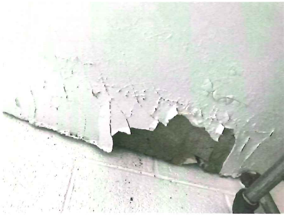
Picture #17: Ceiling damage due to water penetration. Stairwell #5, but this can be found in areas throughout. Especially level 3.
