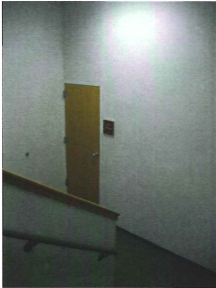
Picture #58: Door swing incorrect. Door to be rated. Wall in which door resides shall meet 1 hour rating. Further investigation would be required.
