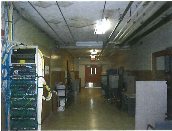
Picture #81: All items removed from corridor, including I.T. Ceiling to be repair or drop ceiling to be installed. Any wall and ceiling penetrations to be sealed.
