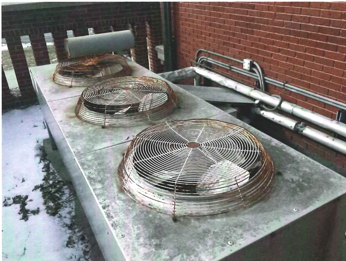
M12 – Computer Room dry cooler
