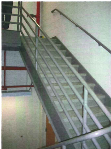
Picture #44 & 45: Stair #1 guardrail not meeting code. No continuous handrail.
