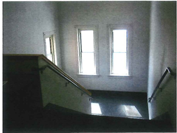
Picture #69 (#70 Sim.): Stair to be enclosed and combustible material replaced. I.E. wall cap, etc. Under a major renovation, code dictates stairs to be enclosed.
