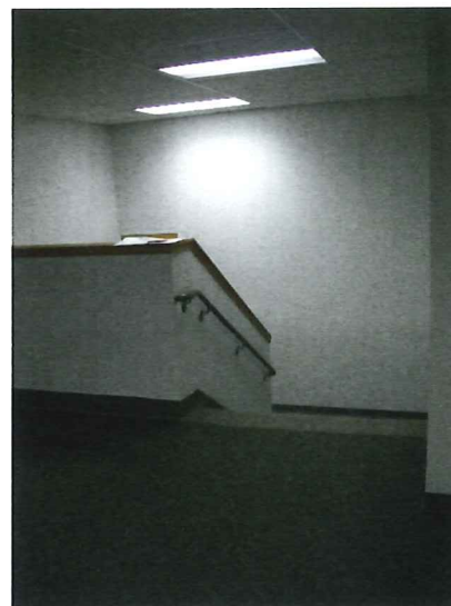
Picture #57: combustible material replaced. I.E. wall cap, carpet, etc. Under a major renovation, code dictates these be replaced.
