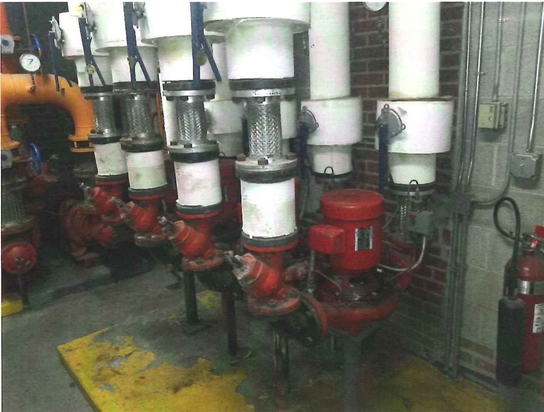
M3 – Heating Hot Water Hydronic Pumps
