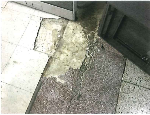
Picture #33: Typical floor remediation required at exposed original terrazzo floor.
