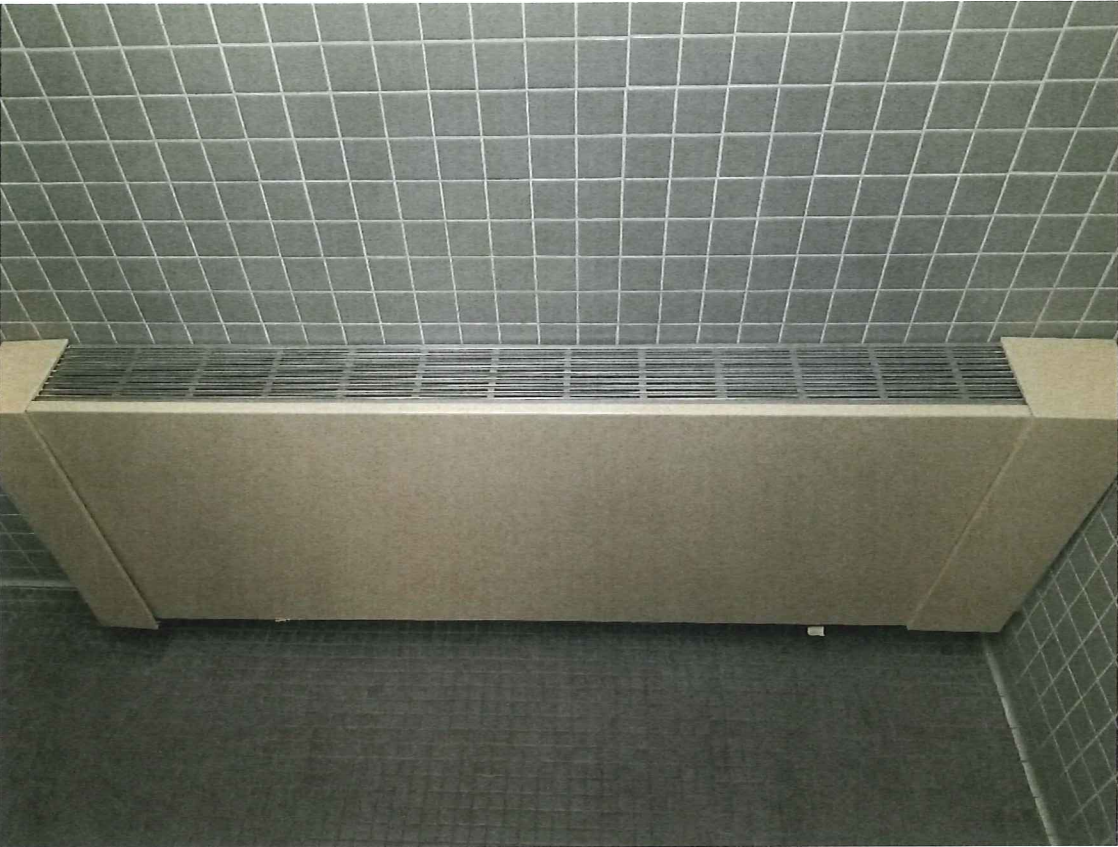
M18 – Fin Tube Radiation
