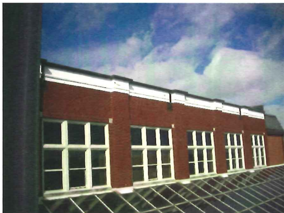
Picture #58: Wood trim peeling paint at the top of the wall.
