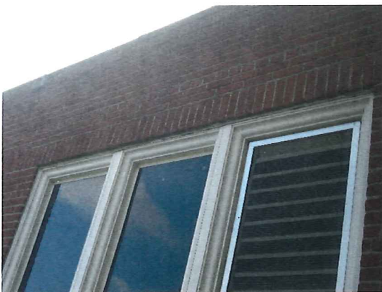
Picture #54 (#55 similar): Typical condition of exterior side of windows. Re-caulk all.
