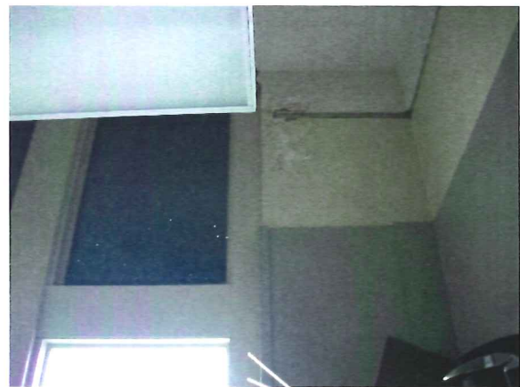
Picture #62: Typical window head on the third level-water damage to window head and wall.
