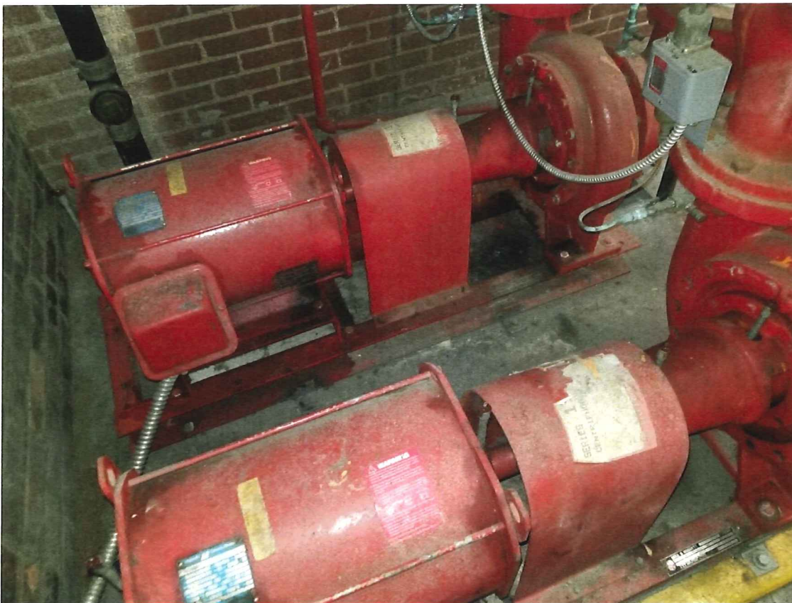
M2 – Heat Pump Loop Pumps
