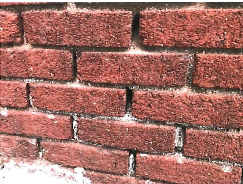
Picture #37: Exterior brick face requiring re-grouting. Limited areas of requirement.
