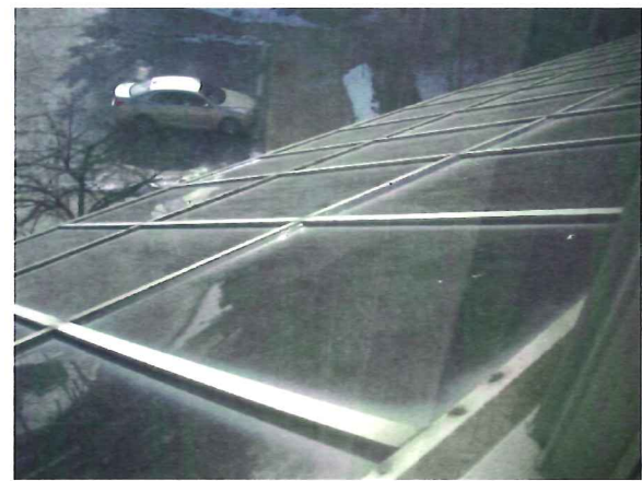
Pictures #48-50: Typical condition of main corridor sloped skylight. Design does not allow for the free flow of moisture.
