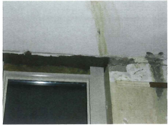
Picture #85: Same water damage at the window head that occurs on level 3.
