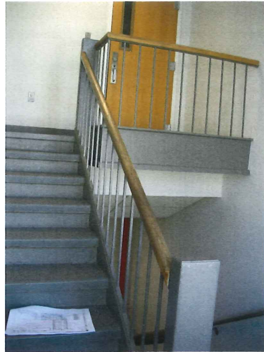
Picture #39: Stair #2-Guardrail not meeting Code. No continuous handrail.
