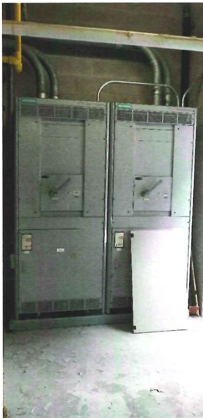
E4 – Main Distribution Switchboard
