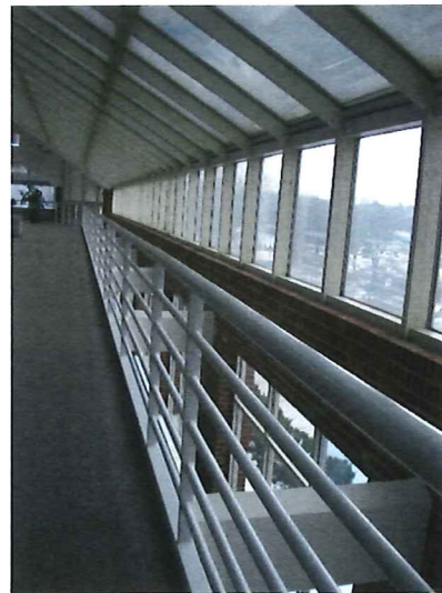
Picture #87: Guardrail does not meet current codes and would require it to be removed and replaced or upgraded to today's codes.
