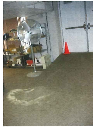
Picture #105: Door requires new weather seals and the surrounding construction be remediated because of damage and weather sealed. In view in the staining due to moisture through the door and door edges.
