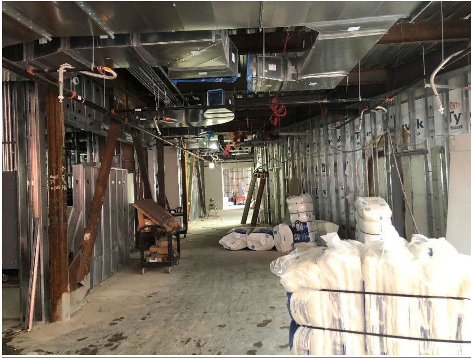
Second floor hallway in Area B where insulation is underway, and MEP is roughed in.
