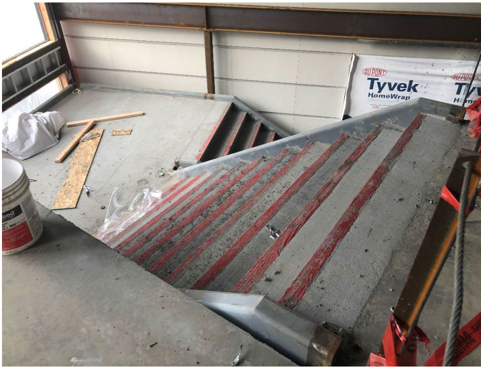
Area B southeast stairway treads with concrete poured and curing.
