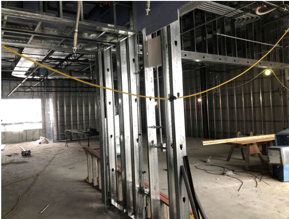
Second floor classroom spaces in the eastern portion of Area B. Very little MEP rough-in has occurred.
