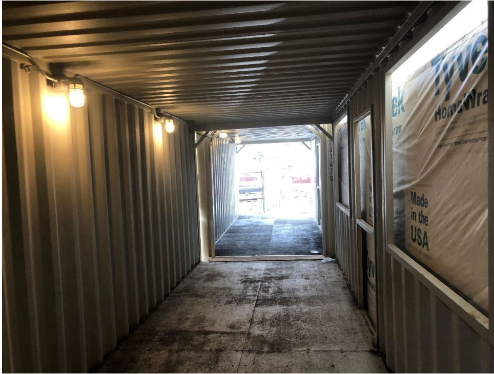
Interior of the pedestrian tunnel protecting the walkway between construction of Areas E and F.
