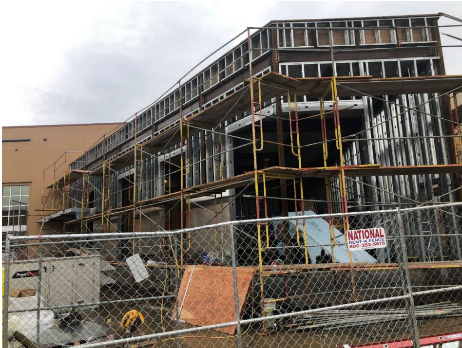
West elevation of Area A (Commons Addition), with walls and parapet framed and roof decking on. Next step is closing in the construction for interior work.
