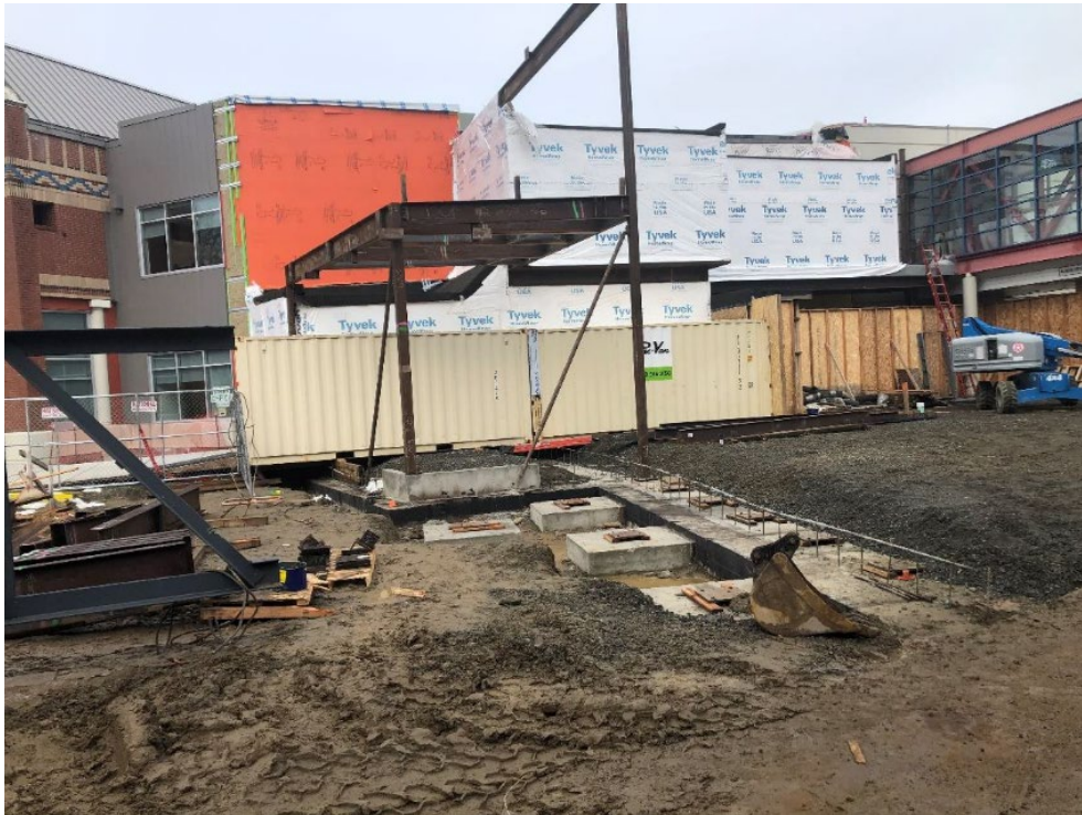
Looking west across Area F footings at Area E. In the center of the photo, a container has been brought in as a pedestrian tunnel for protection from overhead work.
