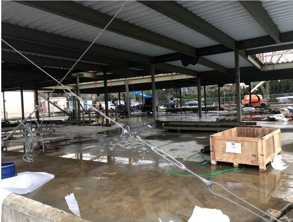
Concrete floor and steel deck ceiling of the first floor of Building B.
