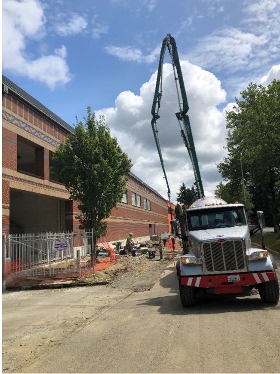
A.1.9. Concrete pumper in action at new foundation area.
