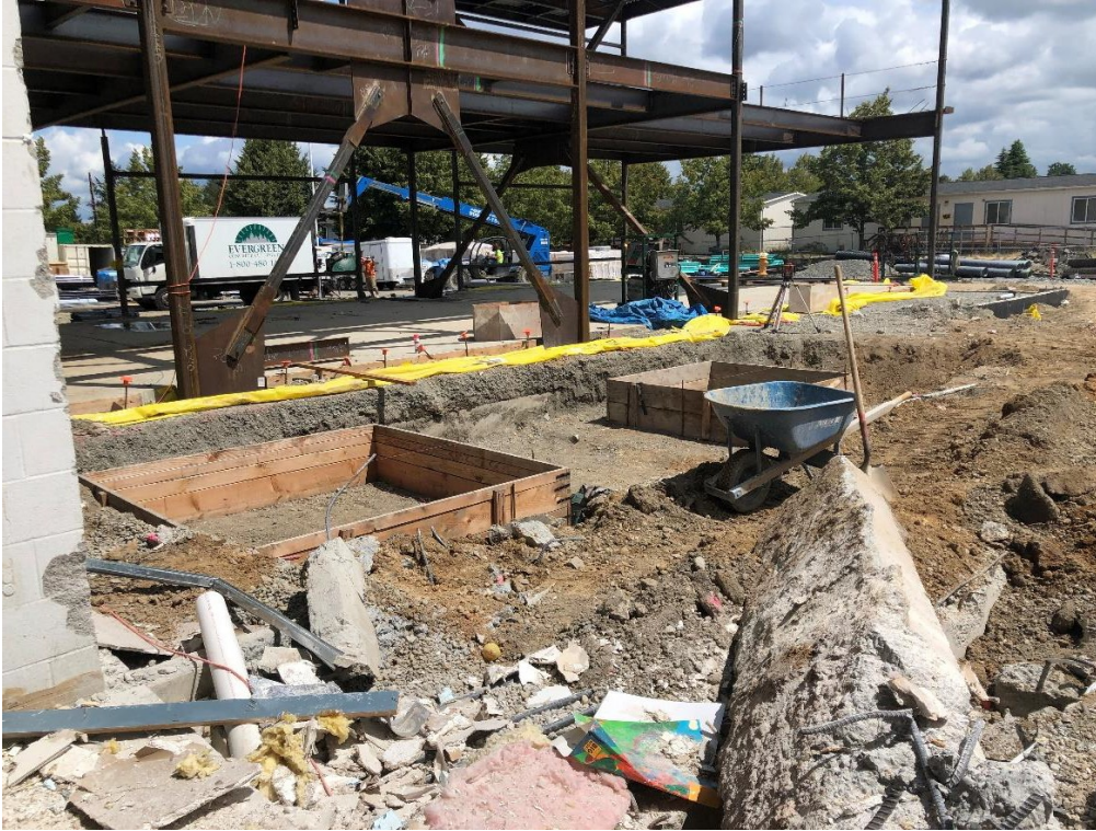
A.1.11. Spread footing forms for new Area B infill.
