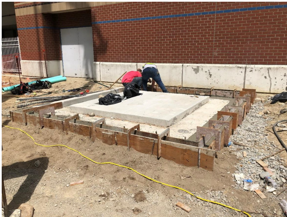
A.1.8. Foundation pad being poured on the south wall of the existing gym/activities wing.
