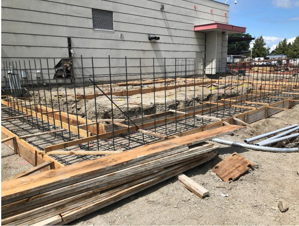
A.1.3. Forming and rebar for the chiller foundation.
