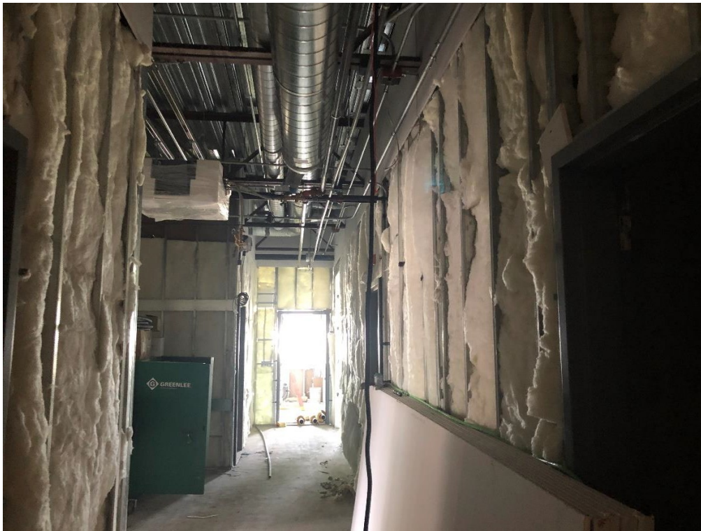
A.1.14. Wall construction insulation in the new administration portion of Area E.
