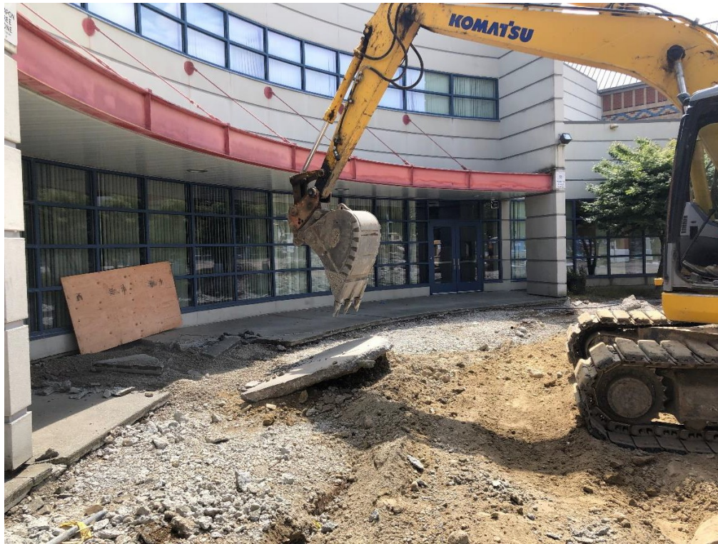
A.1.1. Sidewalk being demolished in front of the lunchroom windows.
