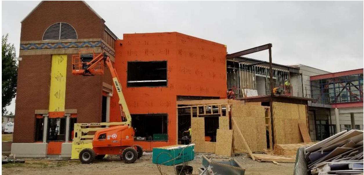
A.1.16. Window mock-up is currently being built. Temporary wood construction walls are being installed at the entry vestibule, temporary roof to follow.
