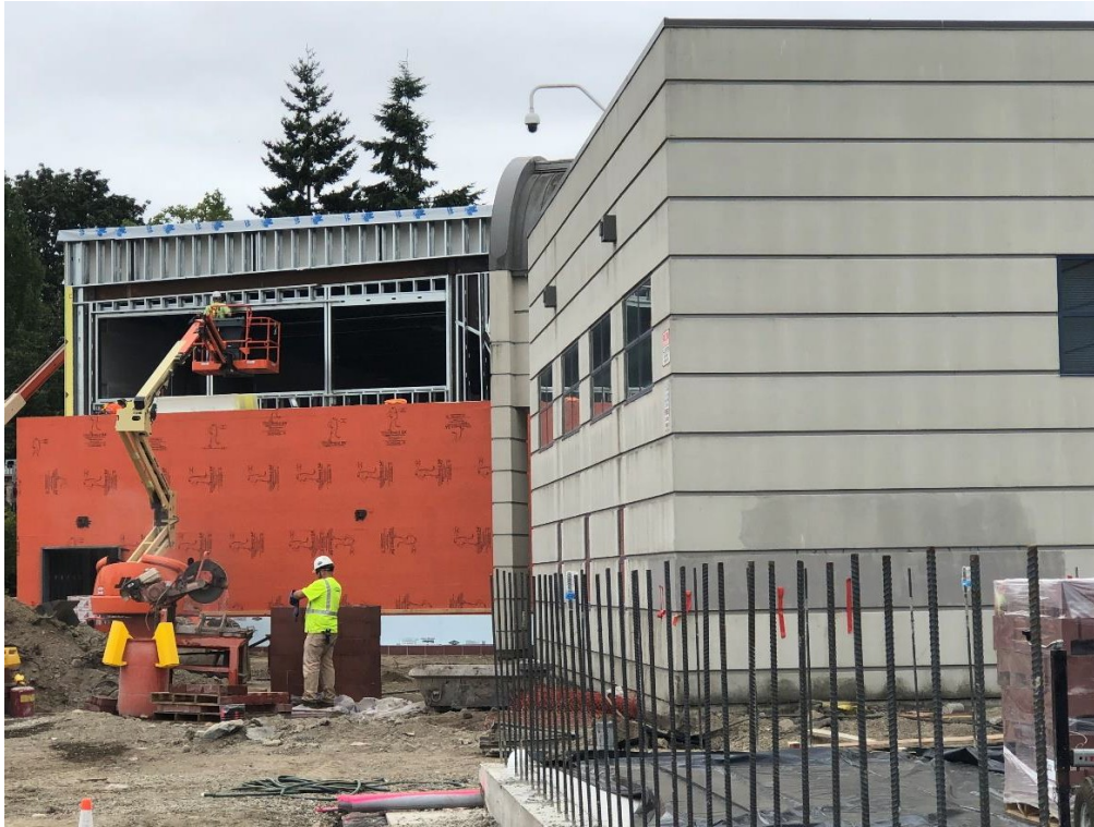
A.1.8. North wall of the new gym (left side of picture) connecting into the existing activity wing. Note that the gym is not yet closed in on the top half.
