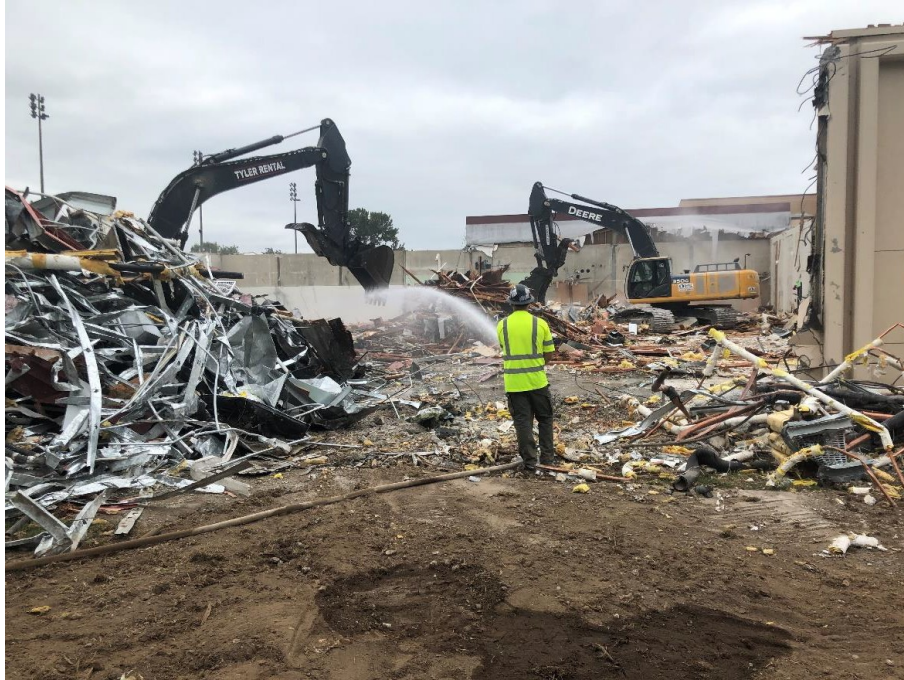
B.1.2. Worker using fire hose for dust control during demolition operation of Building B.
