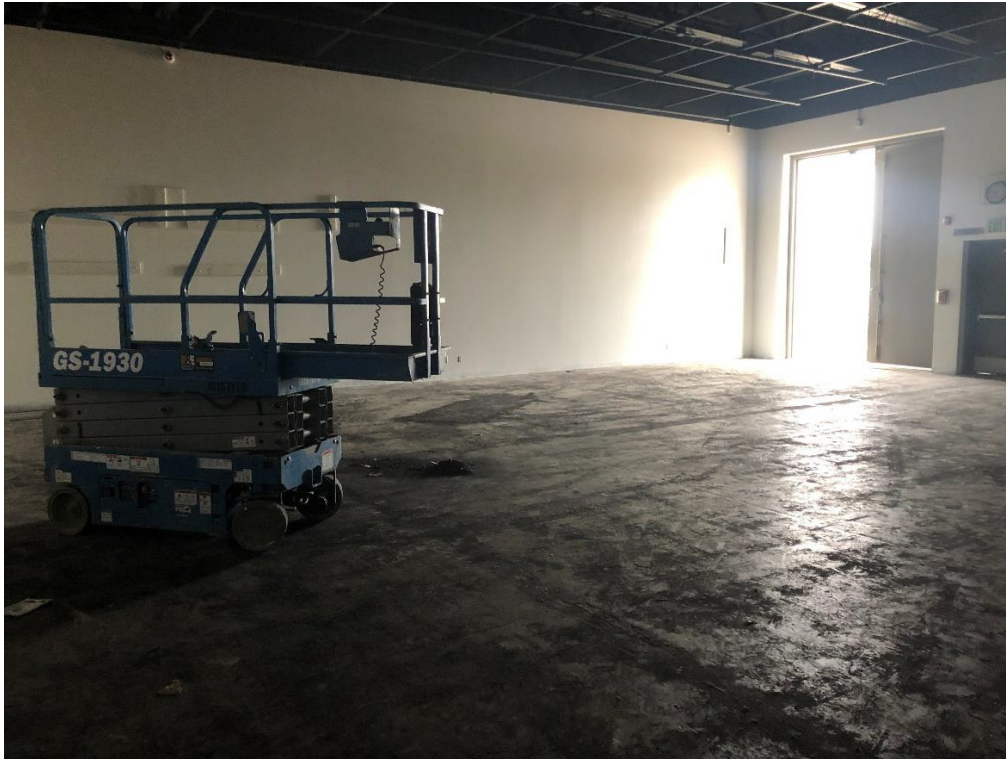
A.1.4. Repurposed weight room, vacated and being readied for a concrete topping slab for supporting weight equipment.
