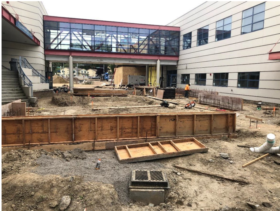
A.1.9. Forms being set for exterior concrete work (seating walls, benches) in the new courtyard area, looking south at the sky bridge adjoining academic wing to activities wing.
