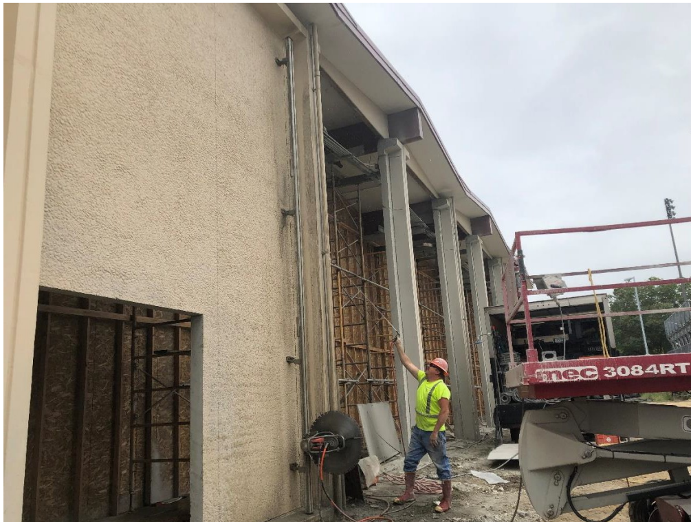
B.1.3. Two full weeks of sawcutting out the concrete wall panels on the west side of the gym. Note the large concrete saw near the sawcutter.
