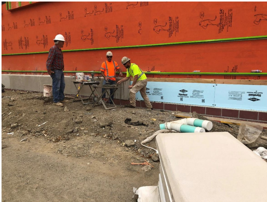
A.1.7. Workers installing lower wainscoting around the exterior of the new gym.
