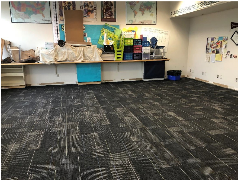
B.1.6. Completed classroom carpeting (typical). Rubber base moulding yet to be installed around the bottom of the walls.
