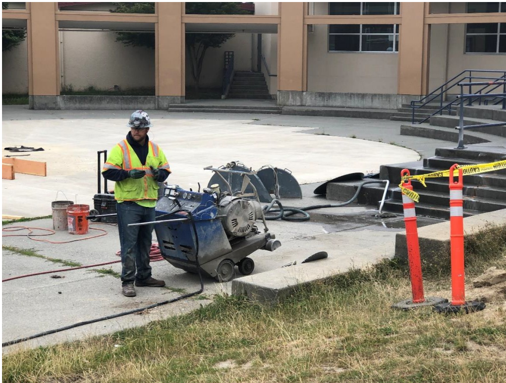
B.1.8. More sawcutting operations. This team is using a much smaller saw to cut the portion of the exterior commons concrete patio that gets removed.
