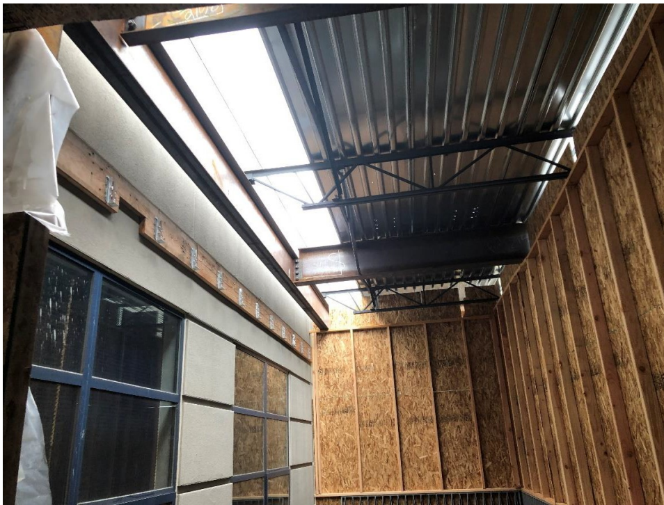
A gap in the roof between the north end of the existing academic wing and the new stairwell being installed for Area A, where rain from last week's significant storm event flooded floors on both levels.
