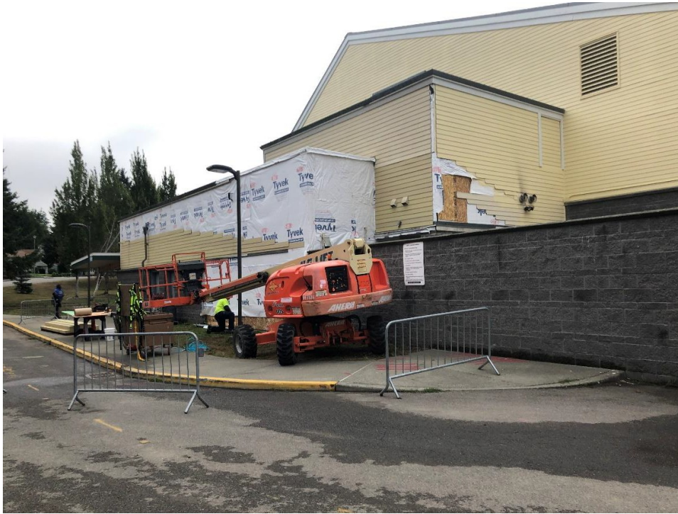
Tukwila: West exterior wall that was rebuilt to alleviate dry rot, now receiving siding and finish work.
