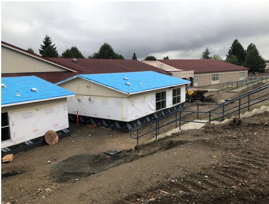
Cascade View: Looking southeasterly across the site of the new modular classroom buildings behind the existing E Wing. These are still under construction, and significant landscape work remains.
