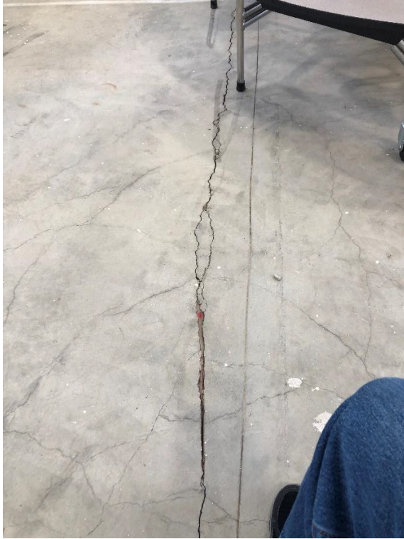
Significant concrete cracking in the floor of the new gym (Area J). This will need to be evaluated for acceptability prior to acceptance. It is unclear if this is a material flaw, or damage from construction equipment.
