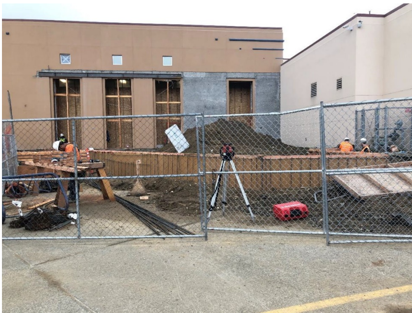
Stem walls being formed for the A Building Commons Expansion area. This construction zone is securely separated from bus drop off zone.
