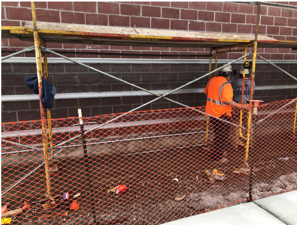
Beginning the process of fascia on the mechanical equipment (chiller) enclosure on the east side of the activities wing.
