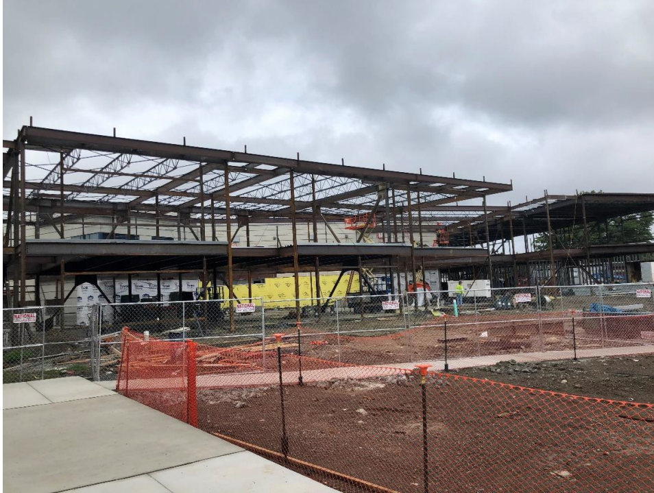
While main emphasis on completing Areas C, E, and J, the steel erection in the Area B/C infill (foreground) and Area A addition (right side background of photo) is progressing.
