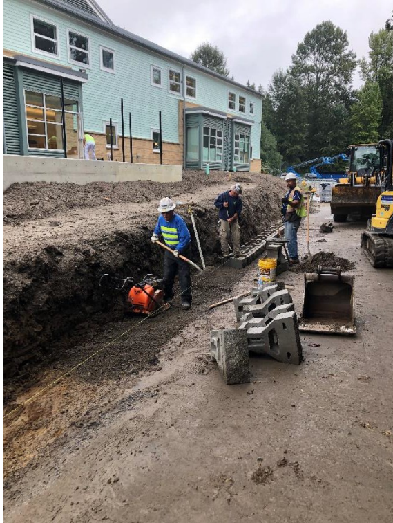
Thorndyke: Looking north easterly at the access road behind the school, where a segmental block retaining wall is under construction.
