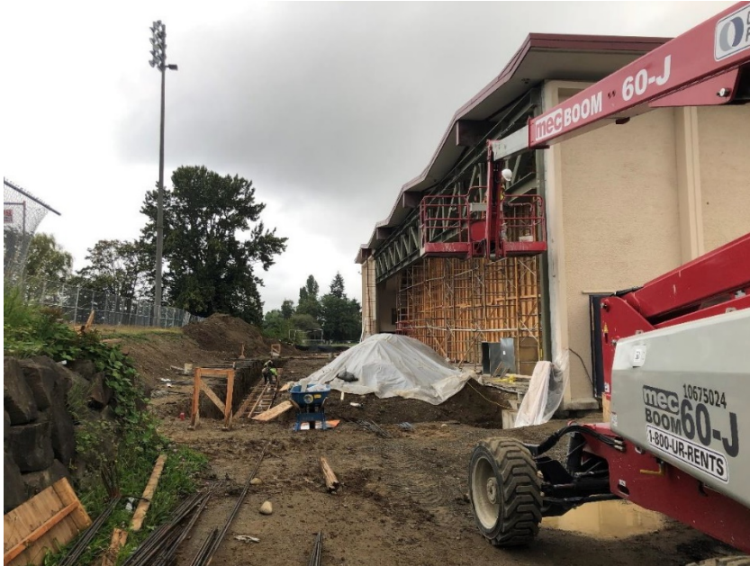
West wall of the gymnasium (looking north), now fully supported on the new girder/truss and support columns. In the left center of the photo, the new strip footing is going into place for the expansion.
