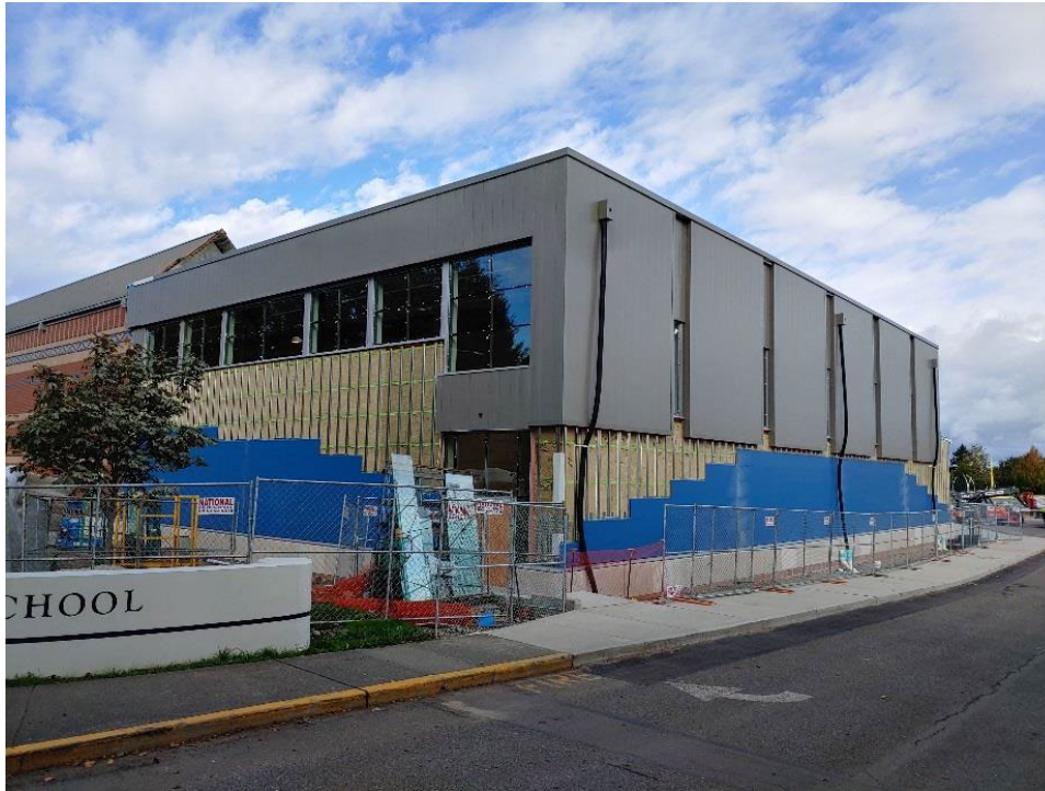
Area J – Auxiliary Gym Addition. Scuppers and temporary downspouts have been installed.
