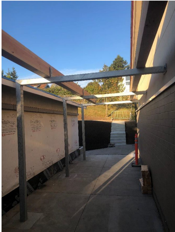
Cascade View: Framing for covered walkway between the west wall of E Wing (right) and the east wall of the new modular (left).
