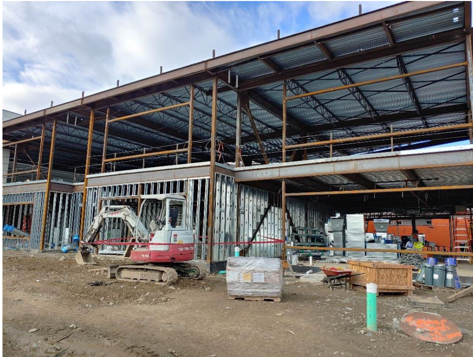
Area B – Steel erection is ongoing. Metal stud framing is ongoing.
