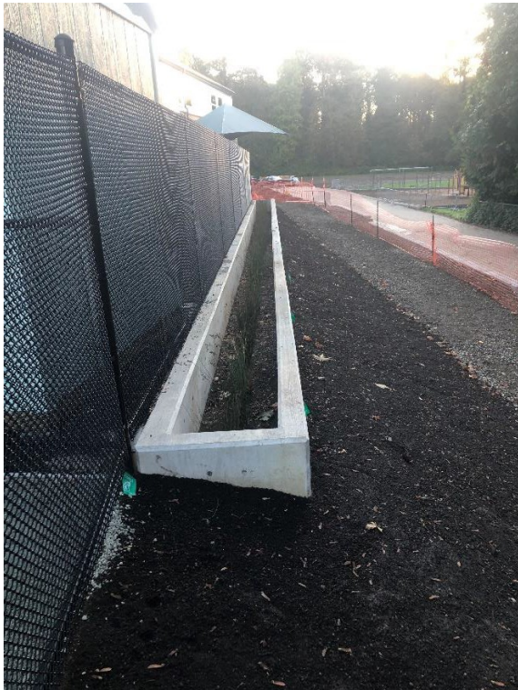
Thorndyke: Bio filtration planter behind Thorndyke now planted and ready for storm water treatment.
