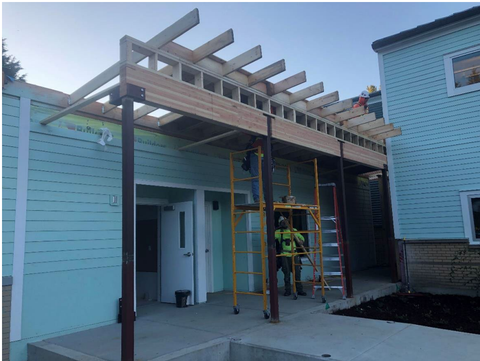
Thorndyke: Framing work progressing on the canopy structure covering the entrance to the new modular building (left), and the causeway to the existing school building (right).
