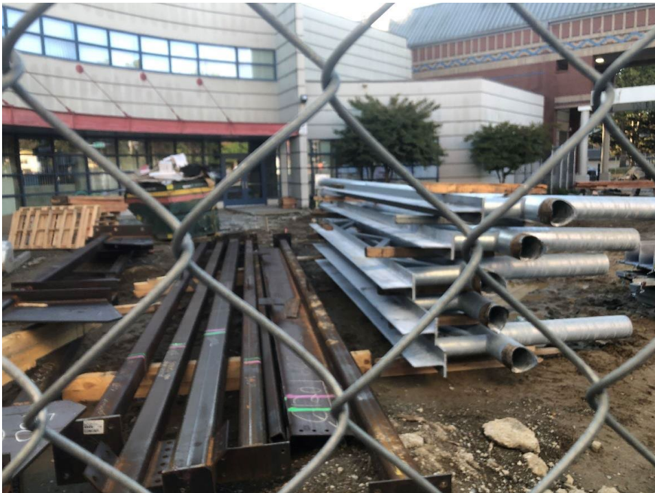
Structural steel that will form space framing in Area F.
