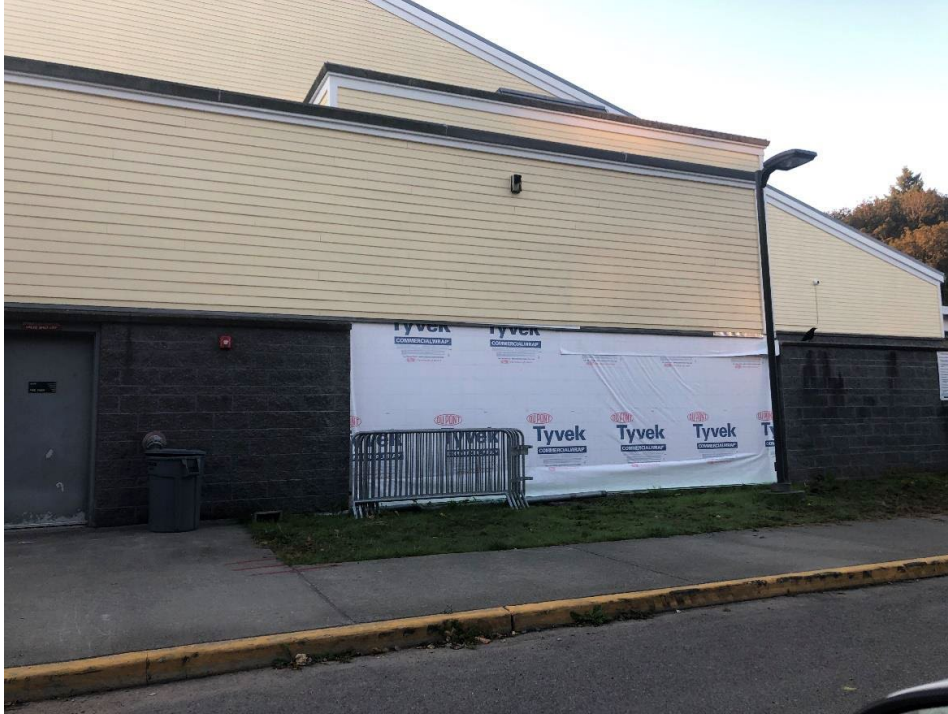
Tukwila: West side of the existing building, where dry rot was discovered during siding replacement. Awaiting replacement concrete block for replacing the façade.
