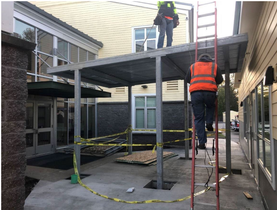
Tukwila: New canopy structure being installed between the new modular classroom building (right), and main school building (left).
