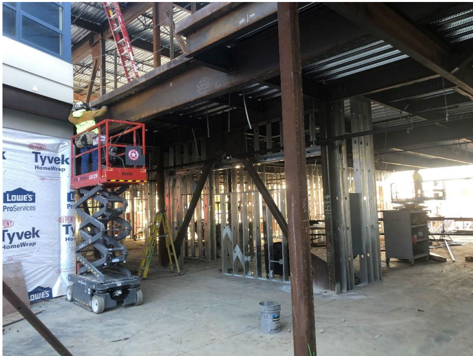
Area B – Welder securing a floor beam in Area B.
