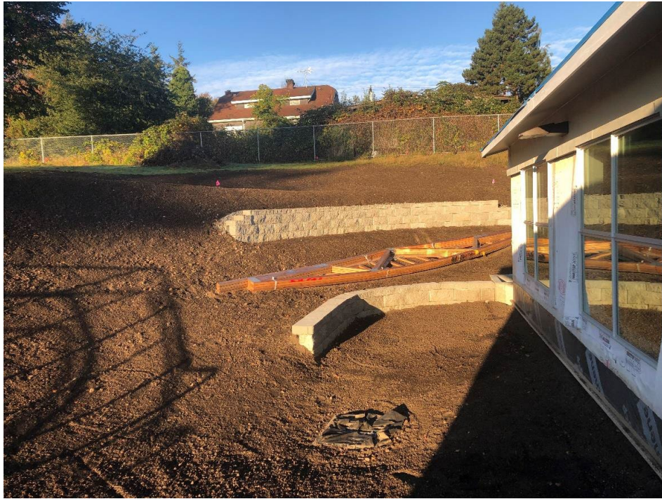
Cascade View: Landscaping progressing significantly. This is the area west of the north modular where short retaining walls have been built, and the fine grading has been completed.
