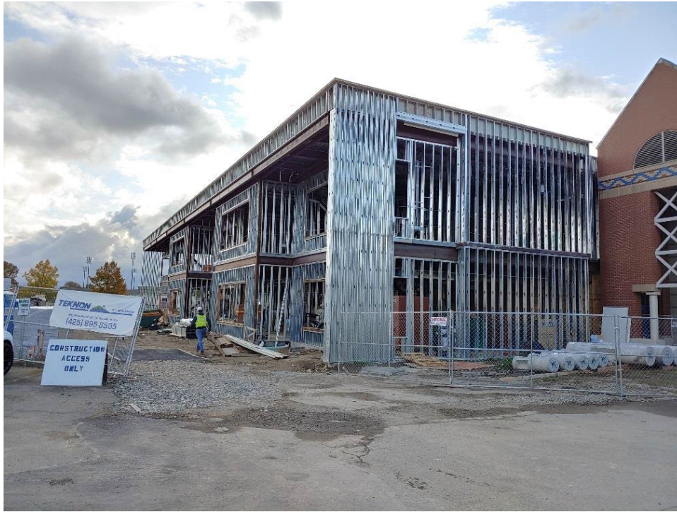
Area A – Metal stud framing is ongoing.
