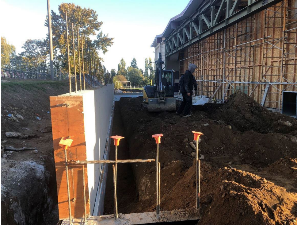
Construction zone for the gymnasium expansion to the west, where walls are now in place and the slab is being readied for a concrete pour.
