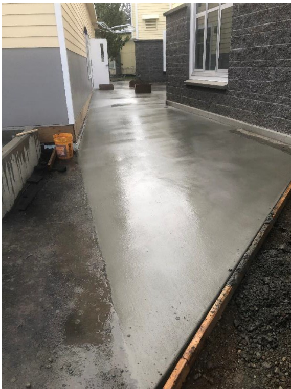
Tukwila: Space between the new modular building on the left, and the existing school on the right, with the concrete slab and sidewalk area poured. A canopy will cover the walkway between the two separate buildings.
