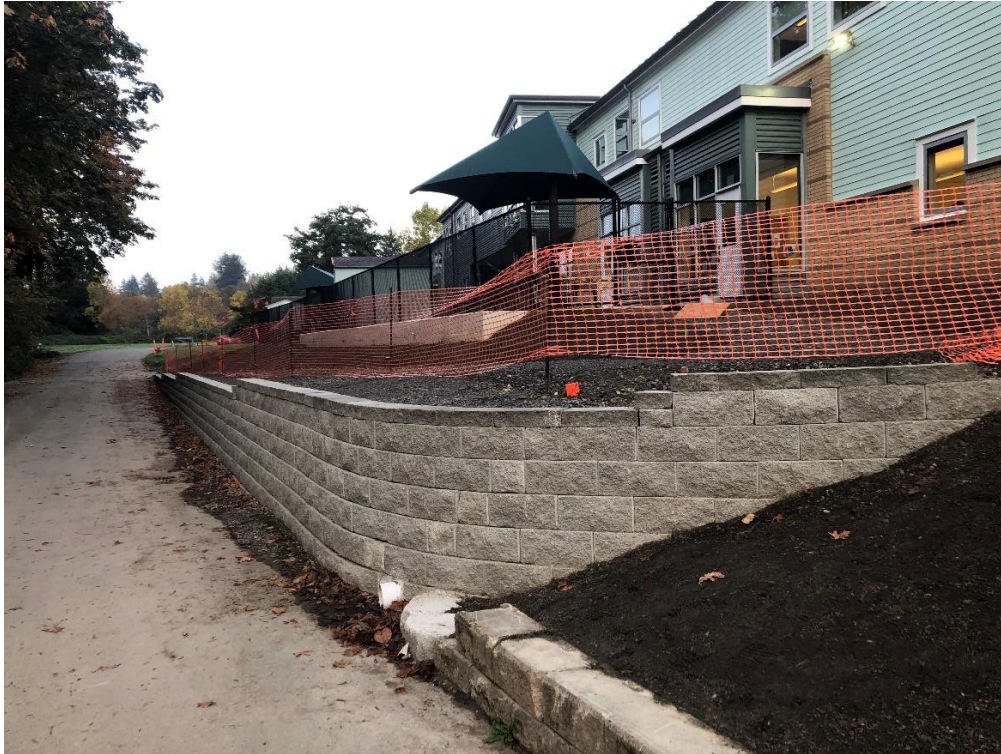
South side of school where a new retaining wall supports the ECEAP playgrounds, new storage Tuff Sheds, and bio filtration units.
