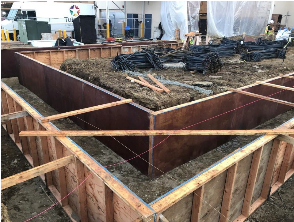
Footing forms in the west portion of the new Building B.
