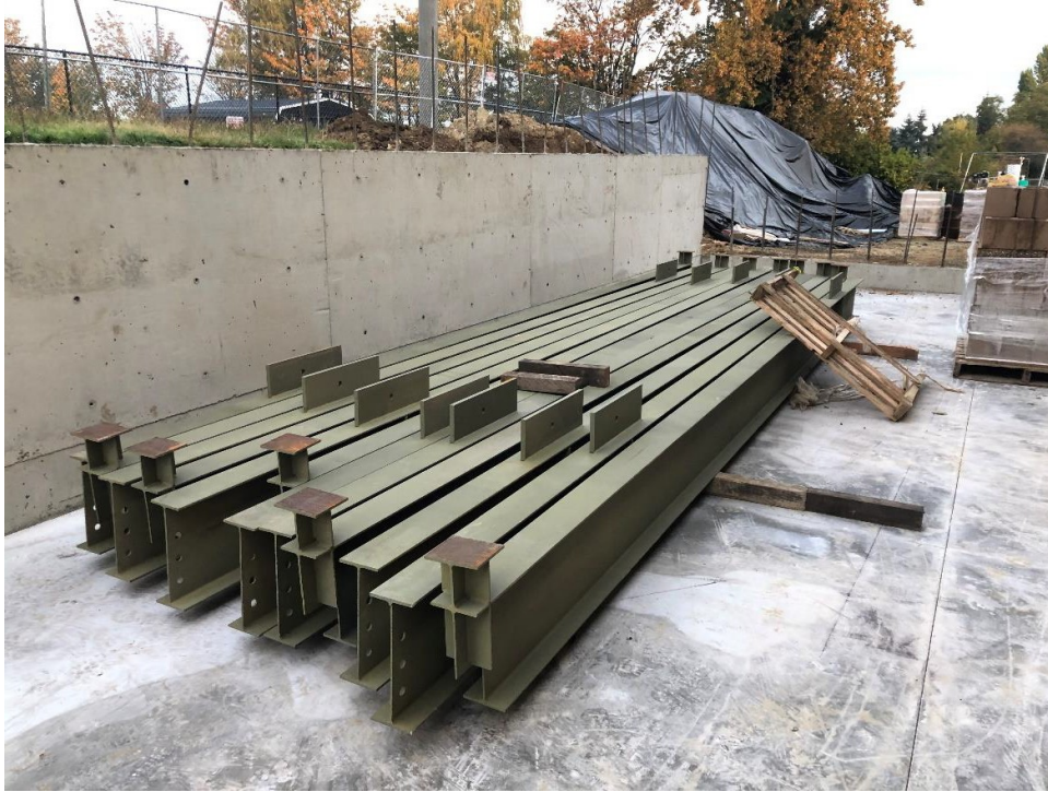
Structural steel for framing the new expansion of the gymnasium (Building C).
