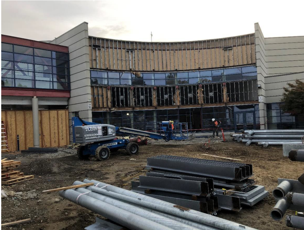
Area F, where the exterior of the existing commons is being demolished.
