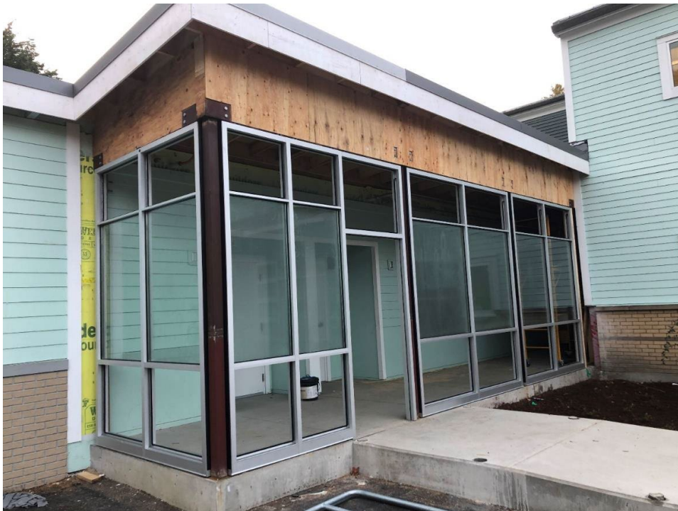
West entrance to new portable classroom, with storefront cover and enclosure nearing completion.
