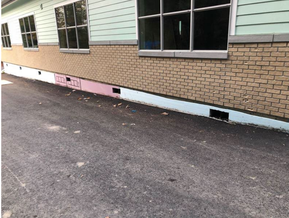
Back (east) side of the modular classroom. Note that skirting is not installed.
