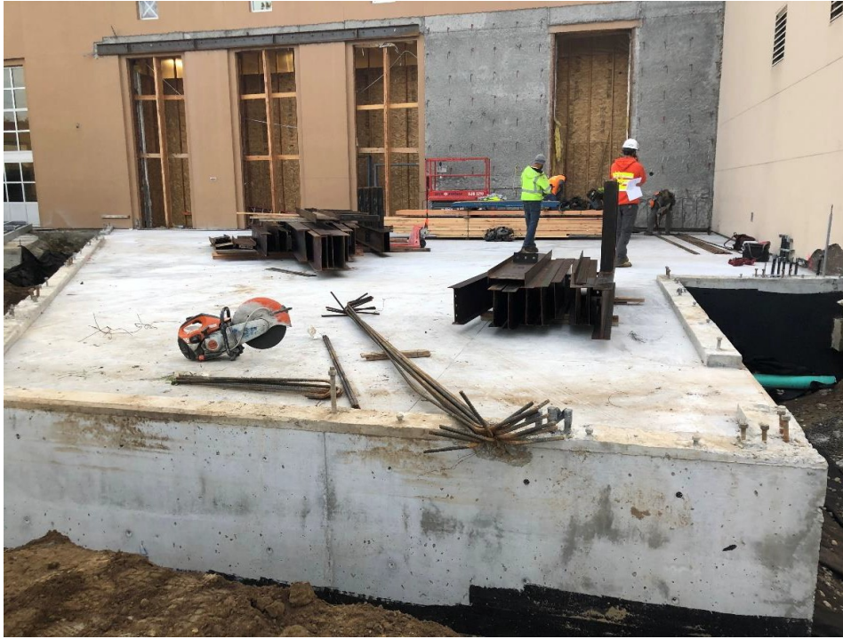
The commons expansion (Building A), where footings and slab are poured, and walls will start now.
