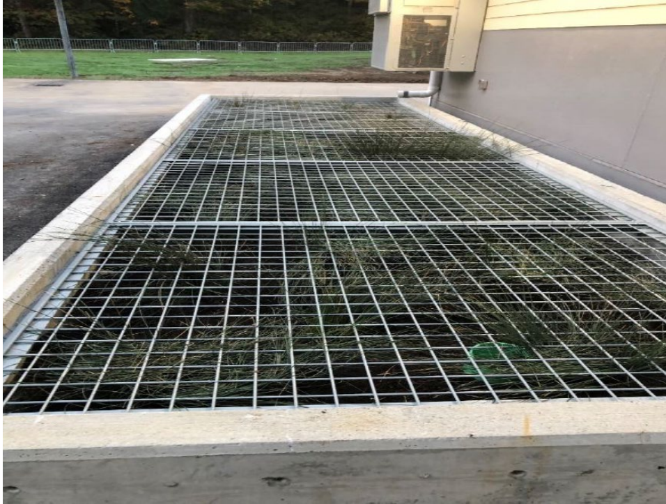
New bio filtration basin that treats storm water runoff.
