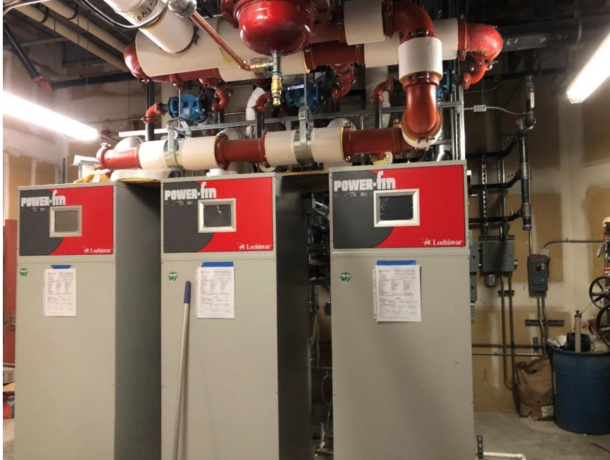
The new boiler units in the mechanical room of existing Building D are completed and ready to begin service.
