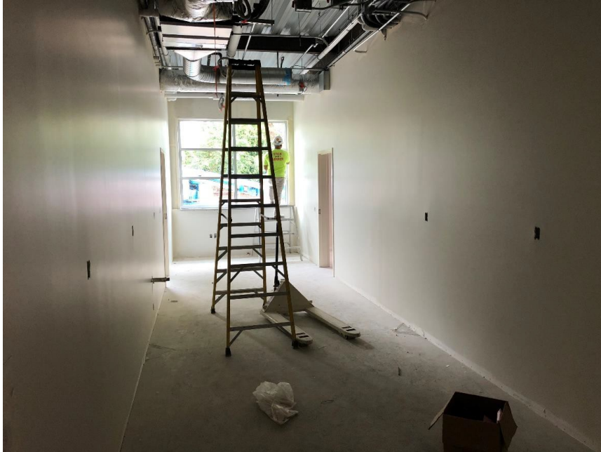
Interior spaces of Building B's ground floor are moving into the finishes phase, with trim being painted around the window frame of this small south facing room.
