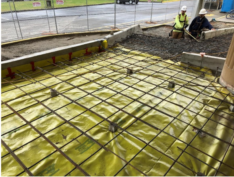
Reinforcement mat being readied for pouring concrete that will become the new slab at the top of the main entrance to SMS.
