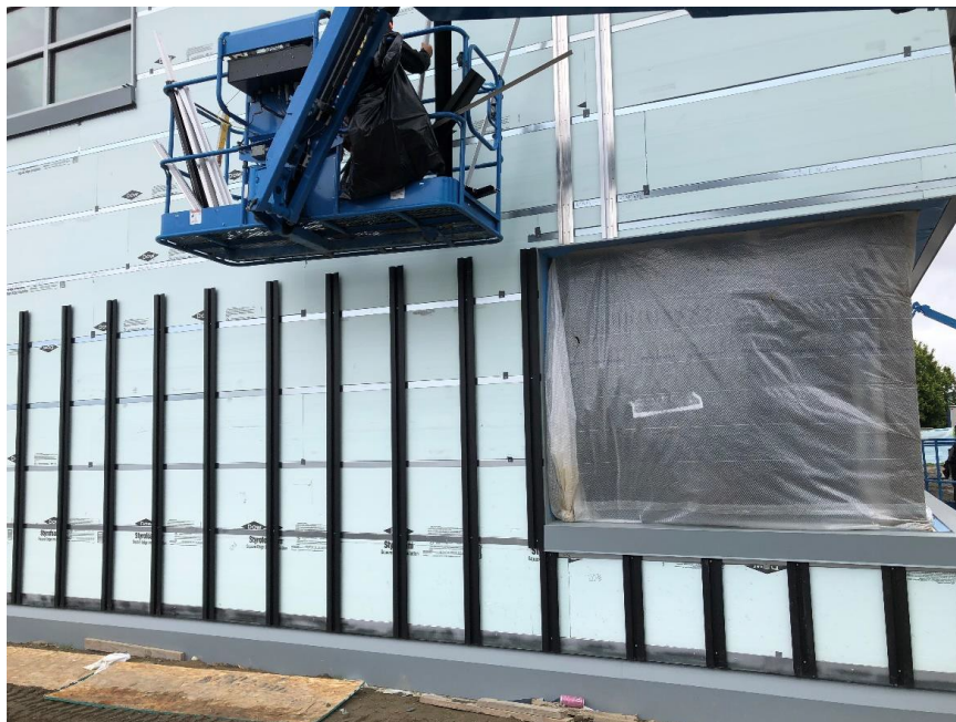
A closer view of installation of the furring, this on the west facing wall, at the southwest corner of Building B.
