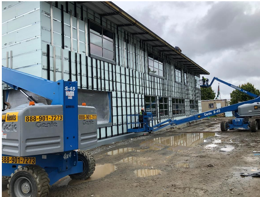
South wall of Building B. Workers are installing furring strips to which the new metal siding panels will be attached.
