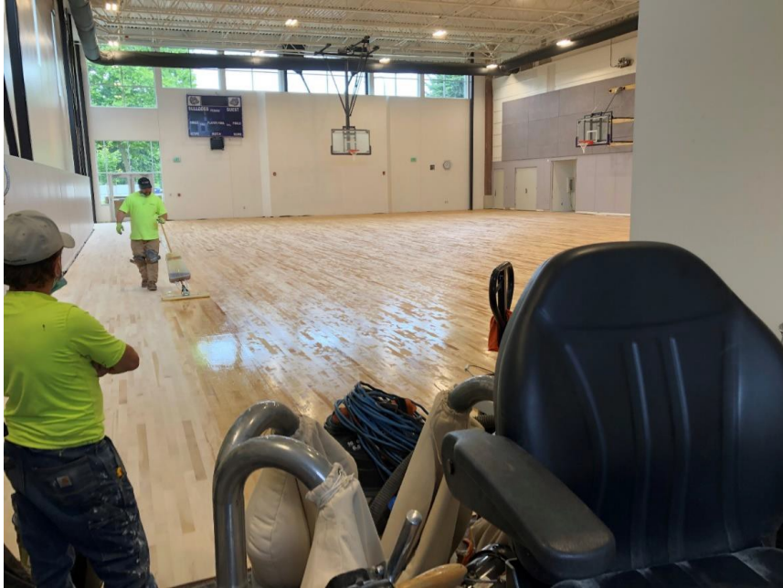
In the new auxiliary gymnasium, installation of the hardwood floor is done, and it is now receiving its surface finishing.
