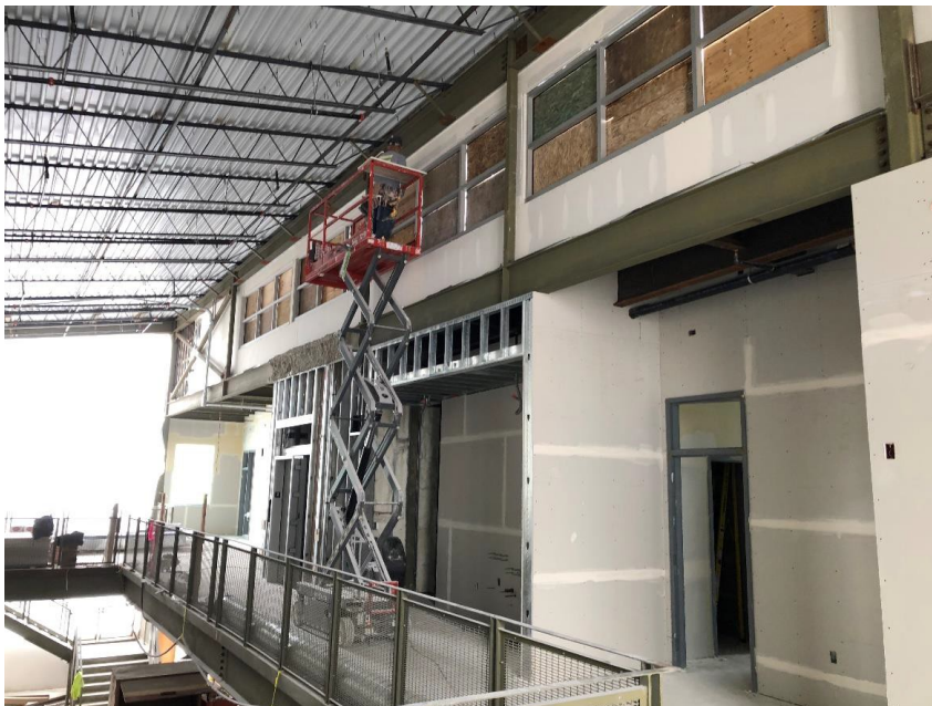
On the upper (second) floor of Building B, most drywall is in. The worker on this scissor lift is trimming out around window frames.
