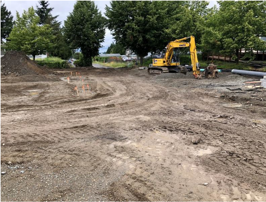
The east end of the new parking lot with staking flags showing where curbing will soon be constructed.
