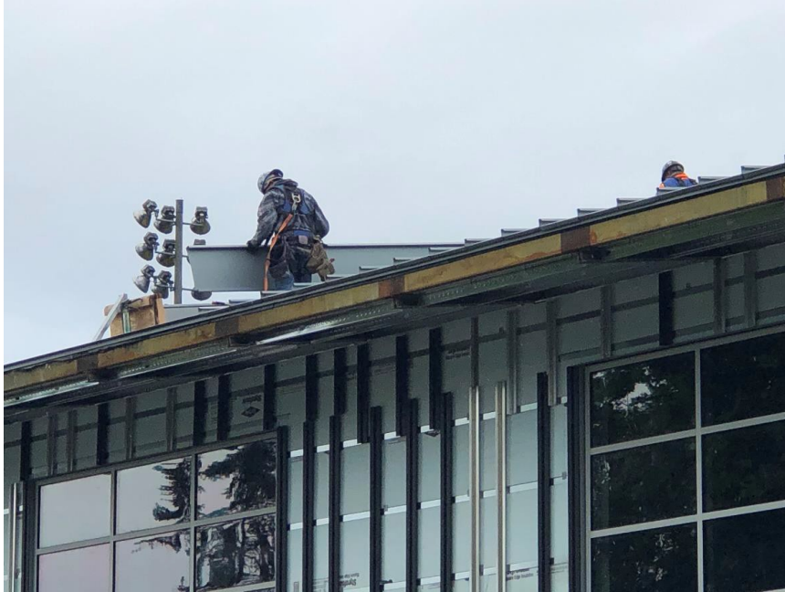
Workers are now installing the metal panel roofing on the low roof (south half) of Building B.
