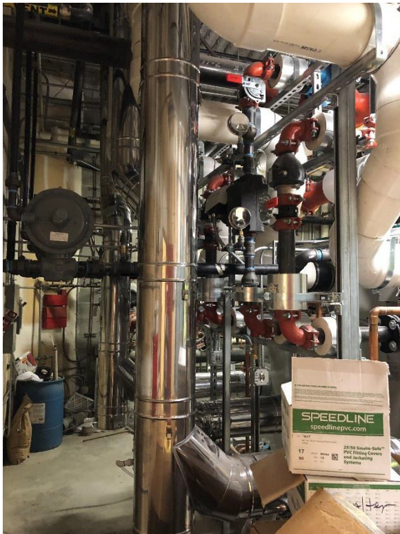
Behind the boilers, a myriad of control valves and systems regulates the fuel to the boilers, water supplies, and heated water, as well as intake and exhaust flues.
