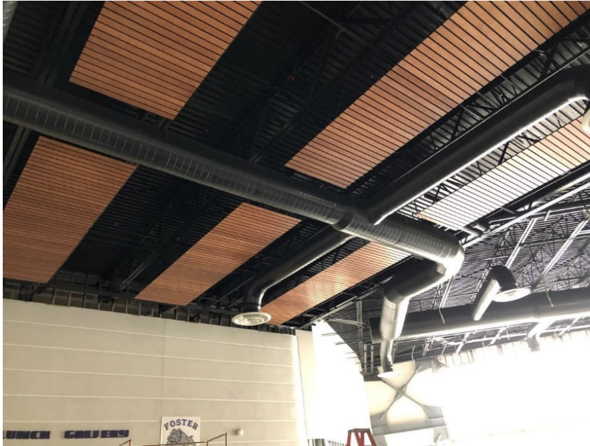
The ceiling of the new Commons with wood slat paneling against the black painted exposed ceiling.
