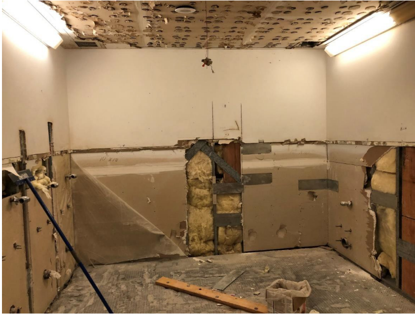
One of the restrooms across from the existing gymnasium, undergoing demolition prior to the remodeling process.
