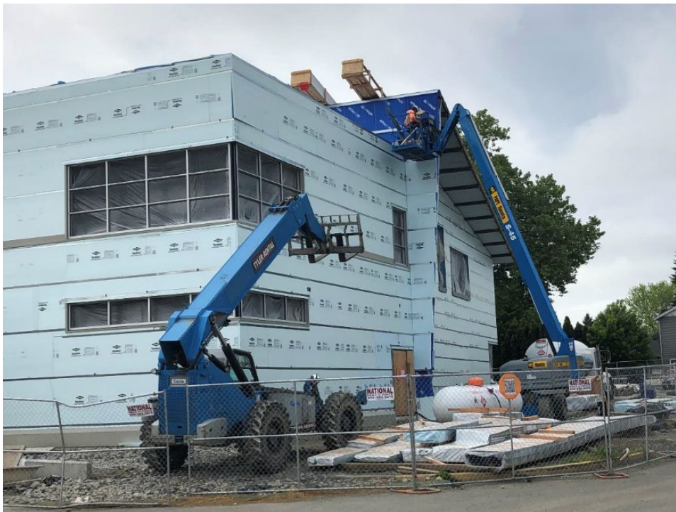
Northwest elevation photo of Building B, workers are heading upward to finish off insulation. Above them, the long metal roof panels, still in their crates hang over the edge of the upper roof area.
