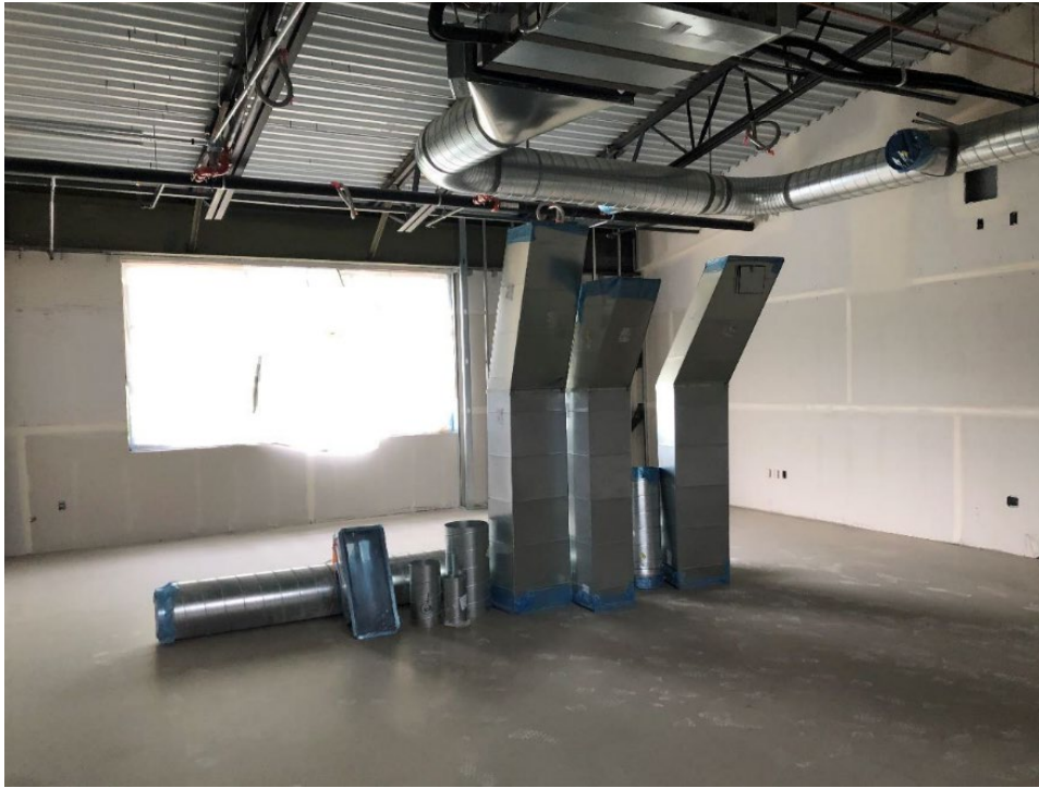
The second floor classrooms are coming along well. This is some of the last mechanical ductwork yet to be installed in second floor classroom ceiling spaces.
