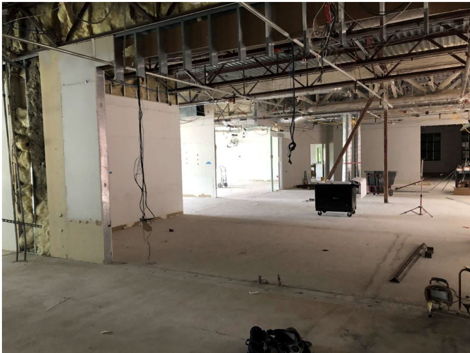
Area C, the selective demolition is complete. When materials arrive, these spaces will all be reconfigured and modernized into new classrooms.
