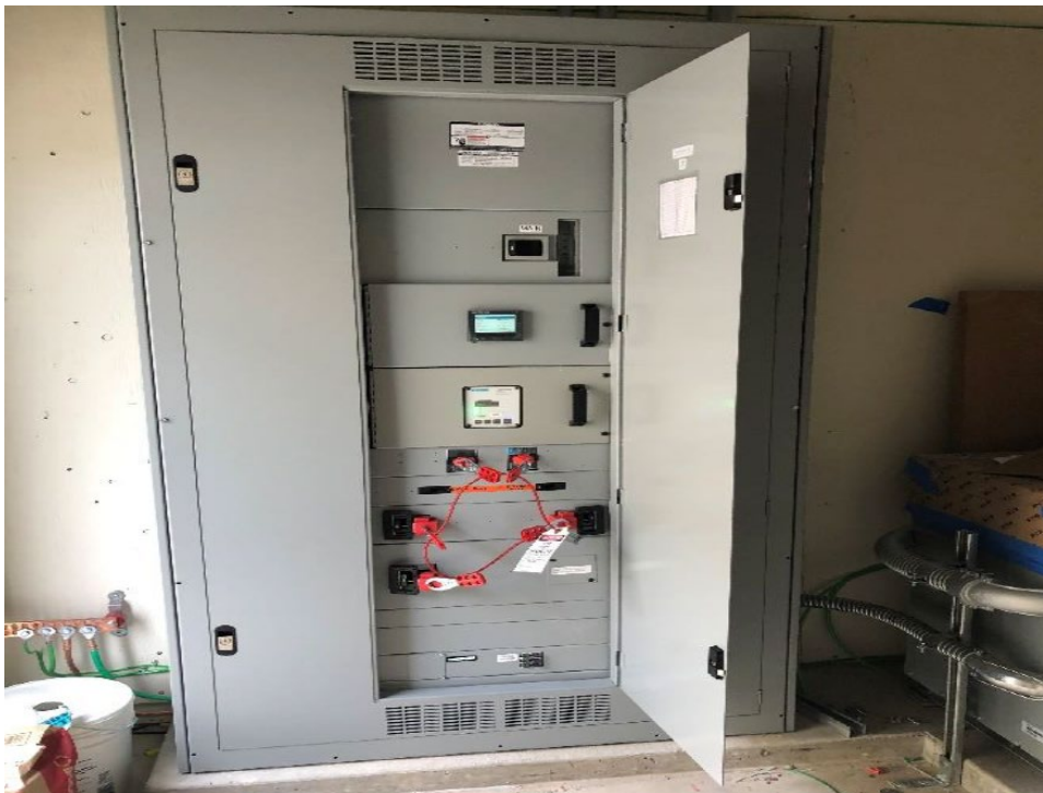
In the utility room, the main incoming electrical panel is housed. Note that the annunciators are operational, signaling that the power is working coming into the new building.
