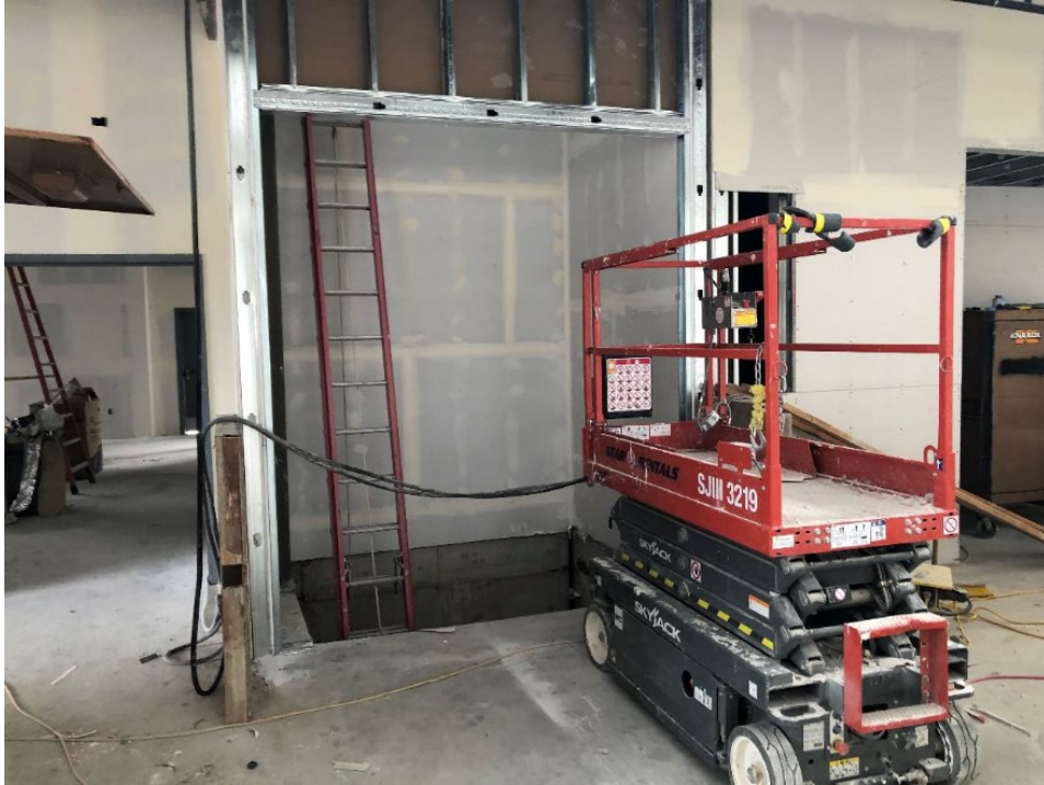
The elevator shaft stands ready for ThyssenKrupp to begin installation of the cab and its hydraulic controls and guides.
