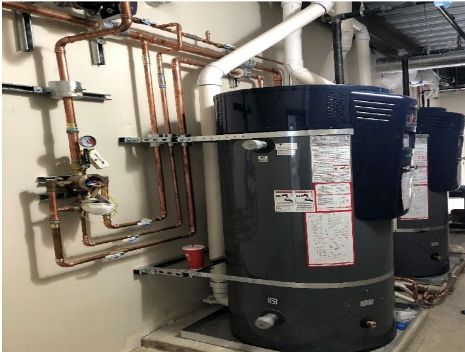
Regulators control the volume, temperature and pressure of hot water being distributed through the building.
