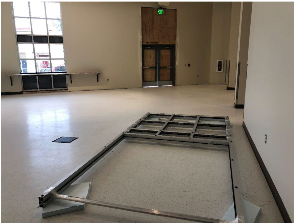
Work is substantially complete in the new Commons Addition in Building A. One of the last remaining items is to install this storefront into the temporarily closed doors in the background of the photo.
