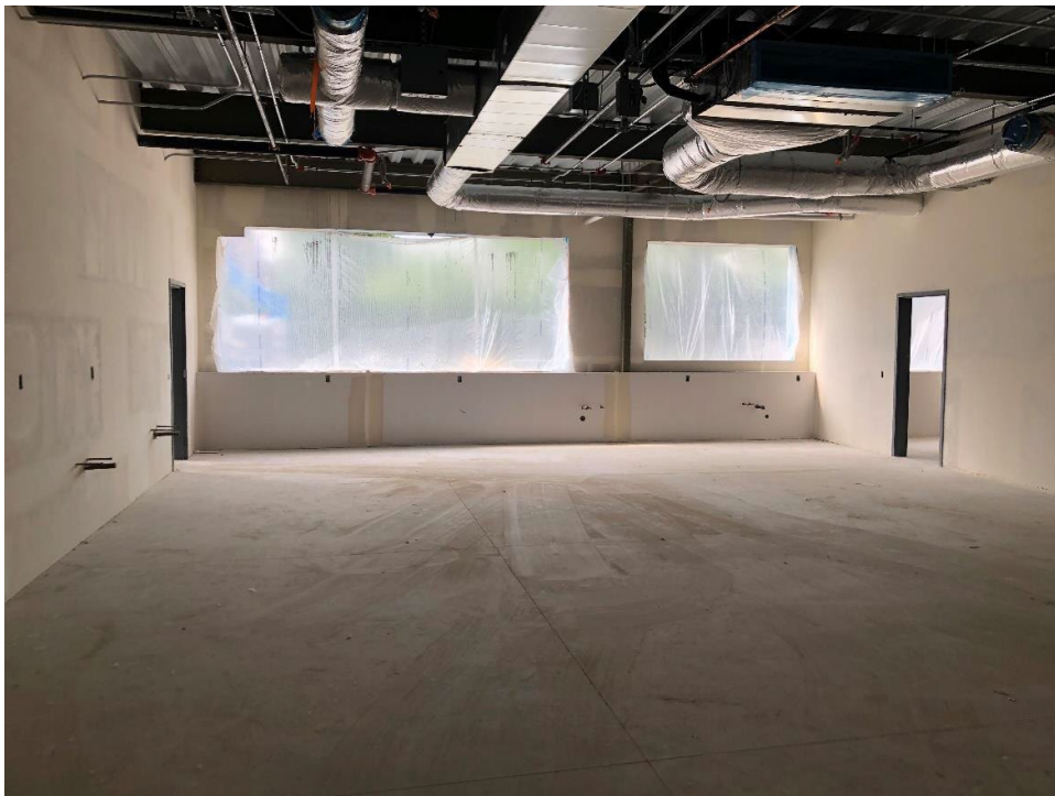
The first floor classroom in Building B now have drywall, with their overhead MEP rough-in work completed. Finishings will now start – windows, floors, ceilings, doors, etc.
