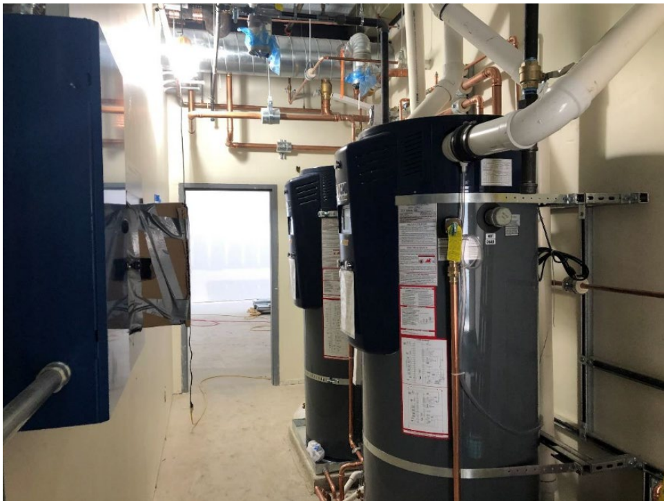
In the Building B mechanical room, large water heaters with intricate copper water lines will distribute hot water through the building.
