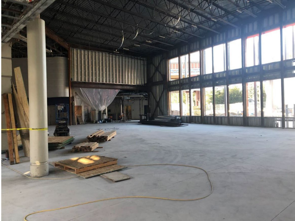
Inside Area F, the concrete slab pours of the floor are now completed.
