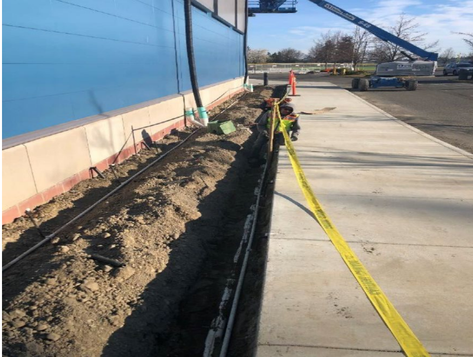
Just outside the east wall of the new auxiliary gymnasium, workers are beginning to install the irrigation systems in the planter strips.
