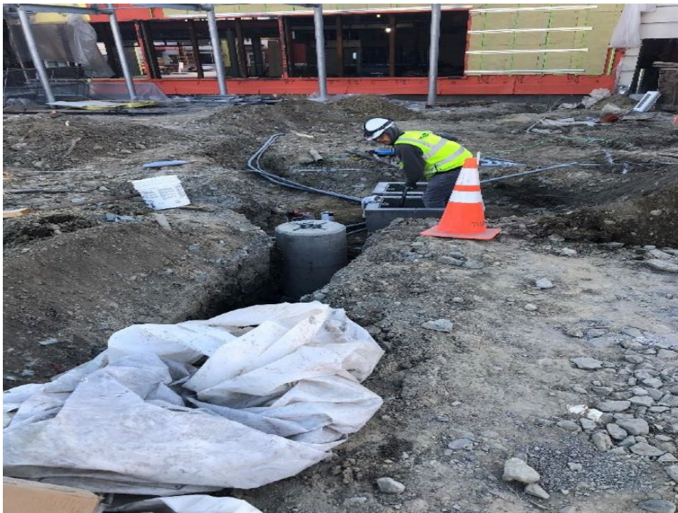
Installing light bases and control boxes outside Area F, in the courtyard portion of Area K.
