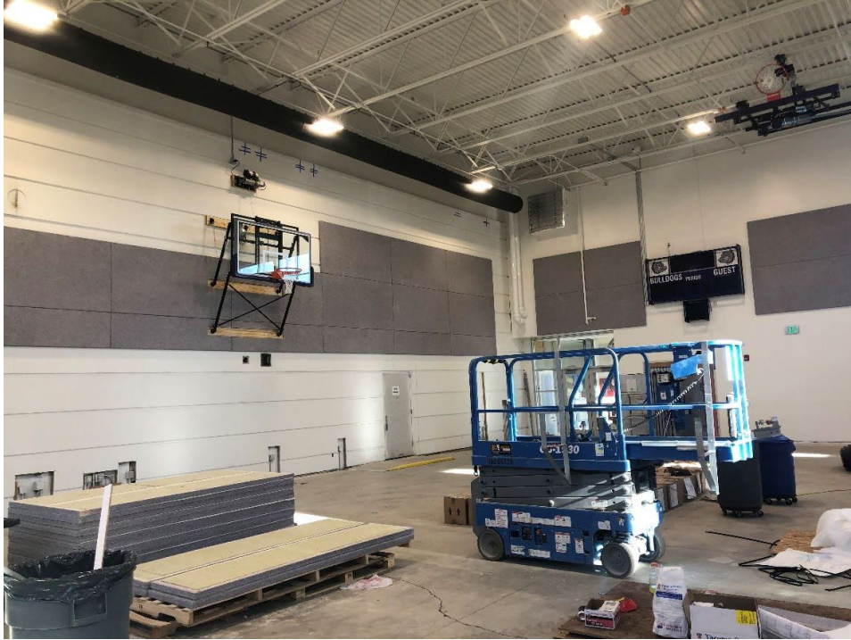
Installing Tectum sound panels inside the auxiliary gym (Area J).
