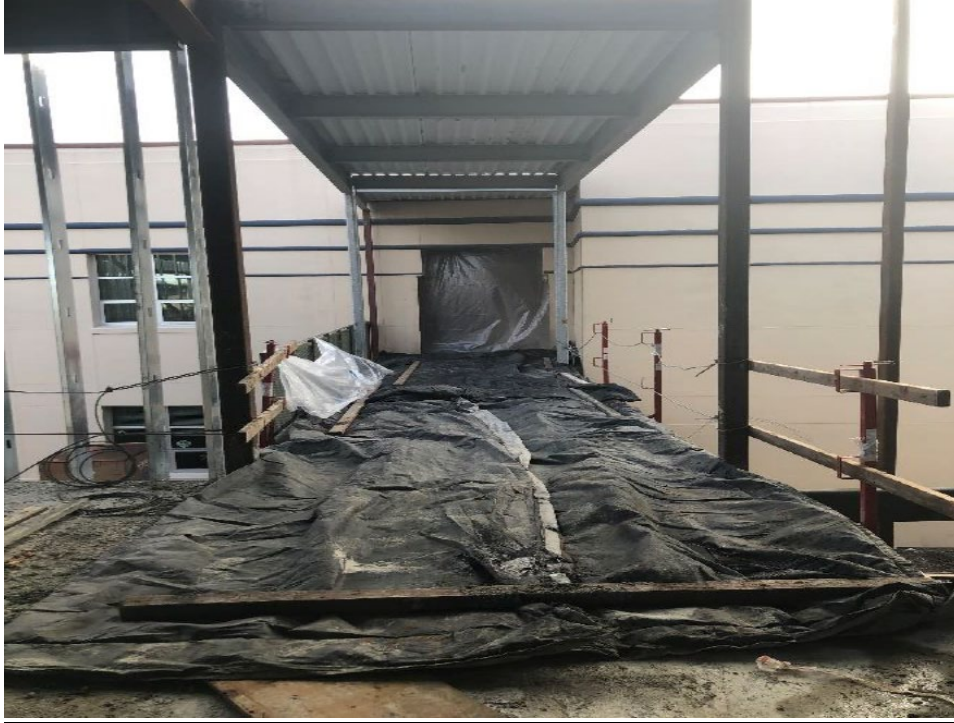
Plastic is covering the newly poured concrete in the sky bridge walkway adjoining new Building B to the south end of Building A (second floor).
