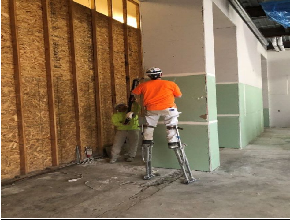
Worker on stilts taping the new columns between the existing and new commons.
