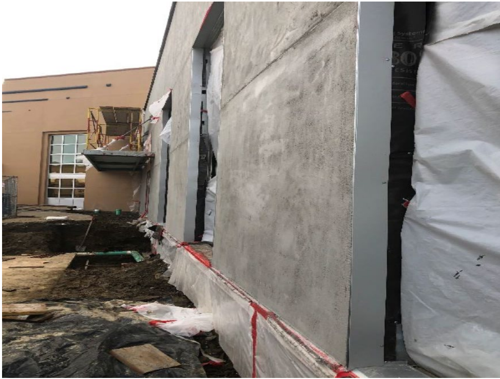
Looking east along the north exterior wall of the commons expansion, showing the composite panels on the walls, and openings for windows.
