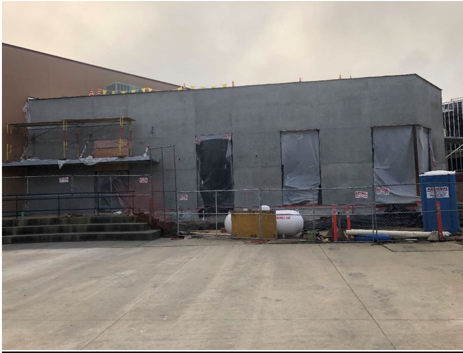
Northwest elevation of the campus additions Area A Commons with exterior wall panels in place
