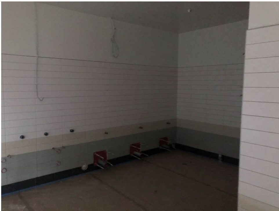
Bathrooms have tile on walls, with floors and fixture to follow.
