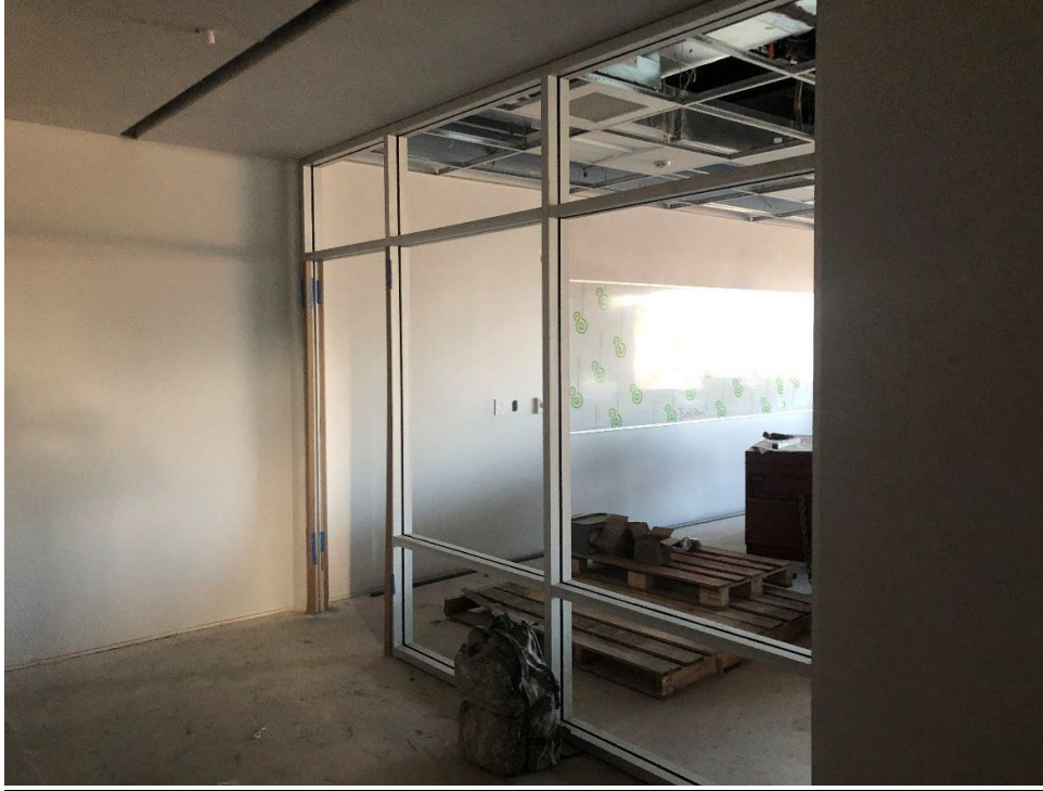
Storefronts and glazing have been installed in Area A Classrooms.
