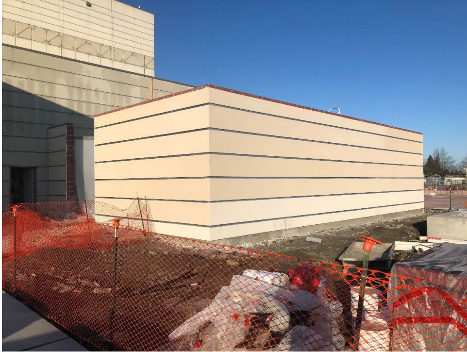
Chiller enclosure with siding completed.
