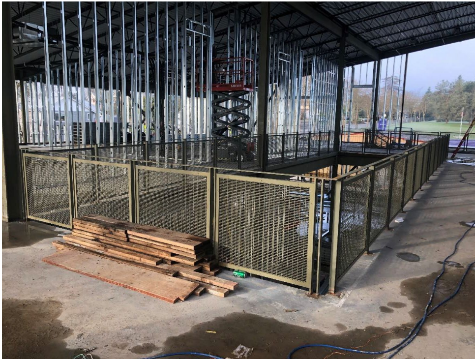
Central open space of second floor of new Building B with newly installed safety railing. The space inside is open down to the first floor.
