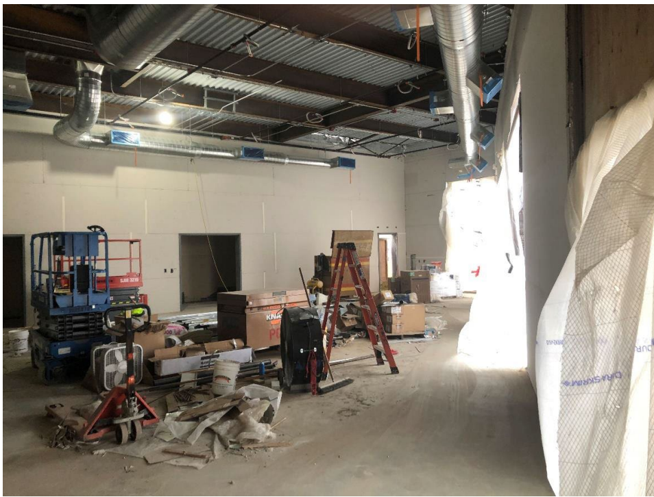
Inside the new commons expansion where interior walls are sheet rocked and the taping process is underway.
