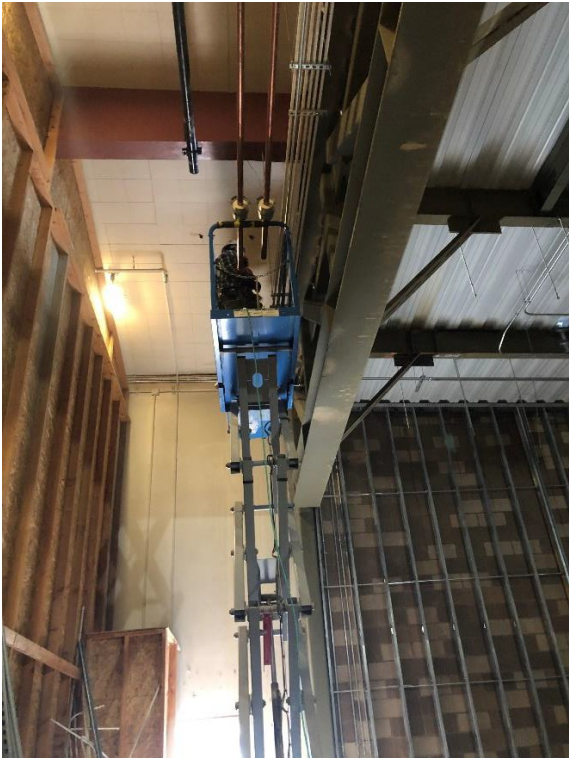
Looking up into the Building G gymnasium expansion, where workers are fitting in the fire suppression system.
