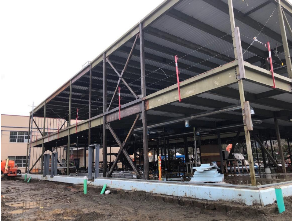
North wall of new Building B, where the low roof decking is shown as complete, and framing will begin soon.
