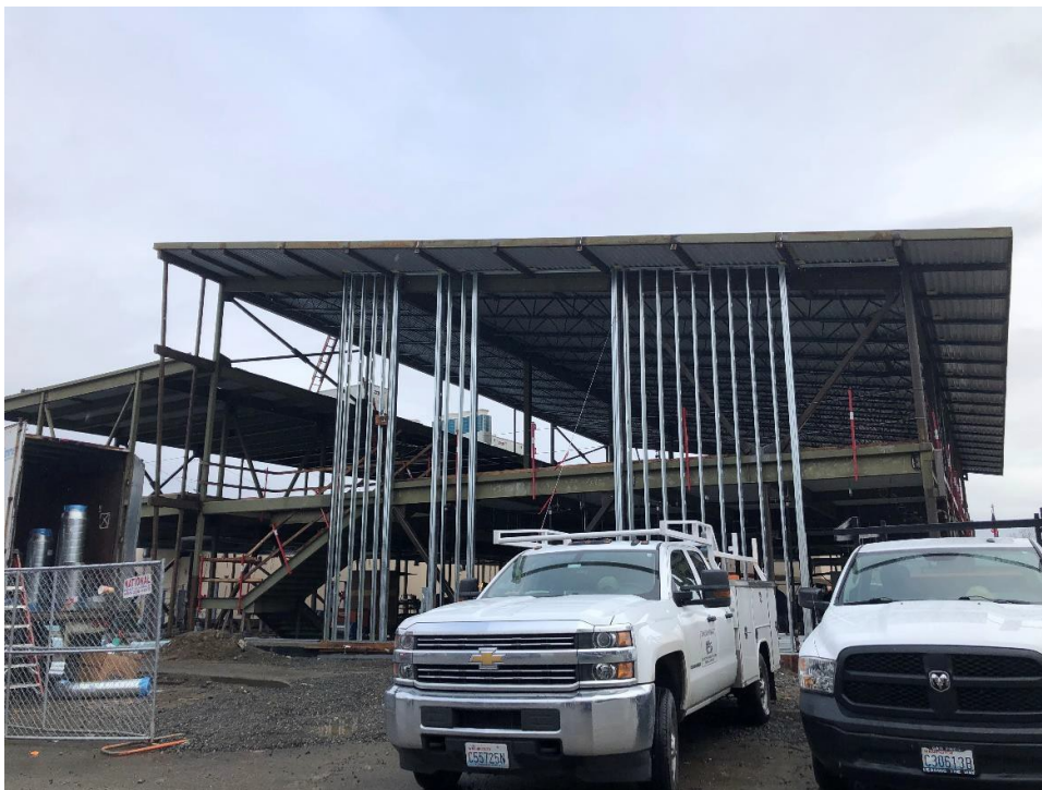
West wall of new Building B, where roof decking is now up and complete, and framing of the exterior walls has started.
