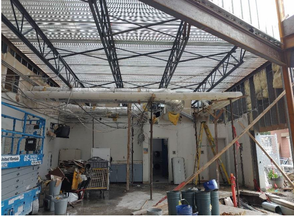
The joists and roof deck have been installed for the small roof at the South end of Area F.
