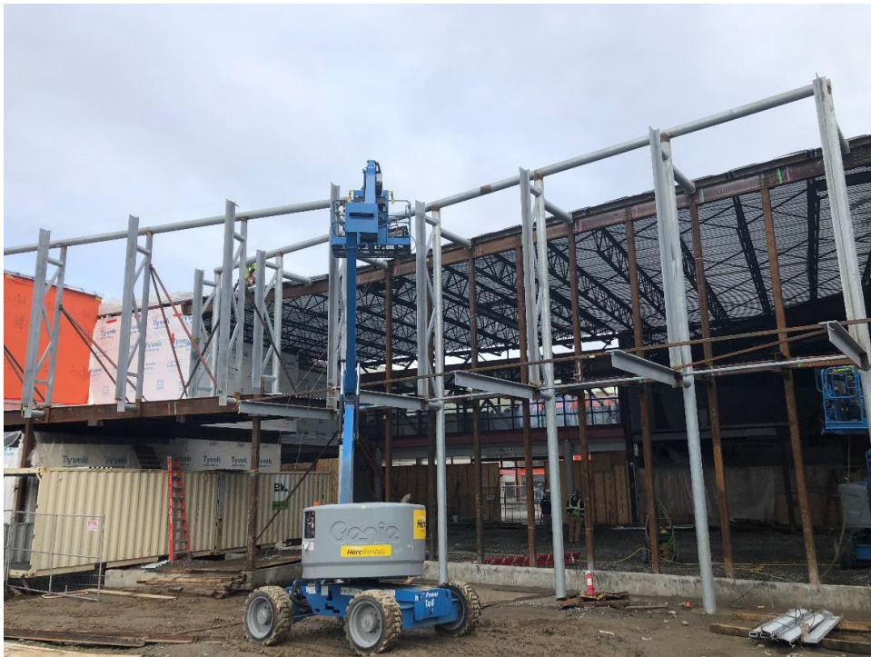
South elevation of the Area F addition and remodeling of the Commons. Steel framing is nearing completion here.
