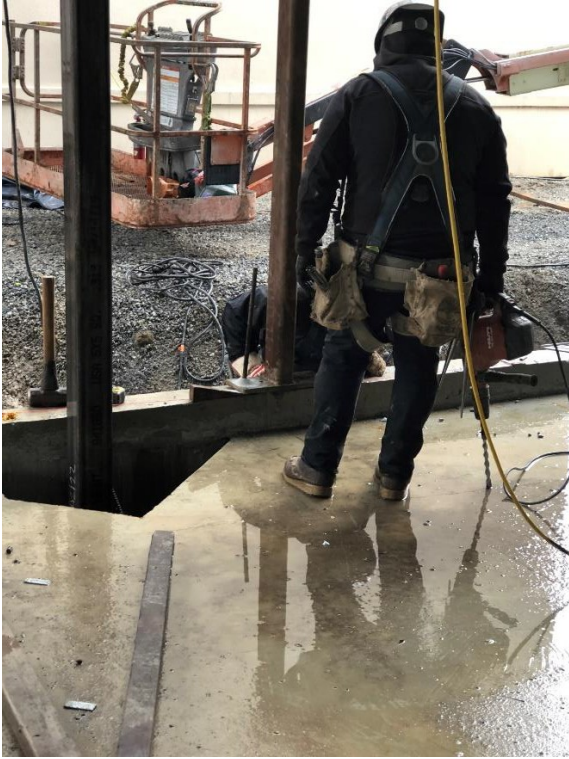
Workers doweling in anchors into perimeter stem wall of Building B.
