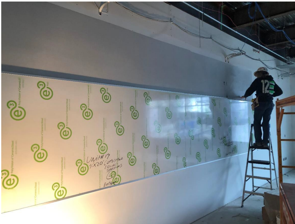
Workers installing vinyl wall covering above installed whiteboards in Area A classrooms.
