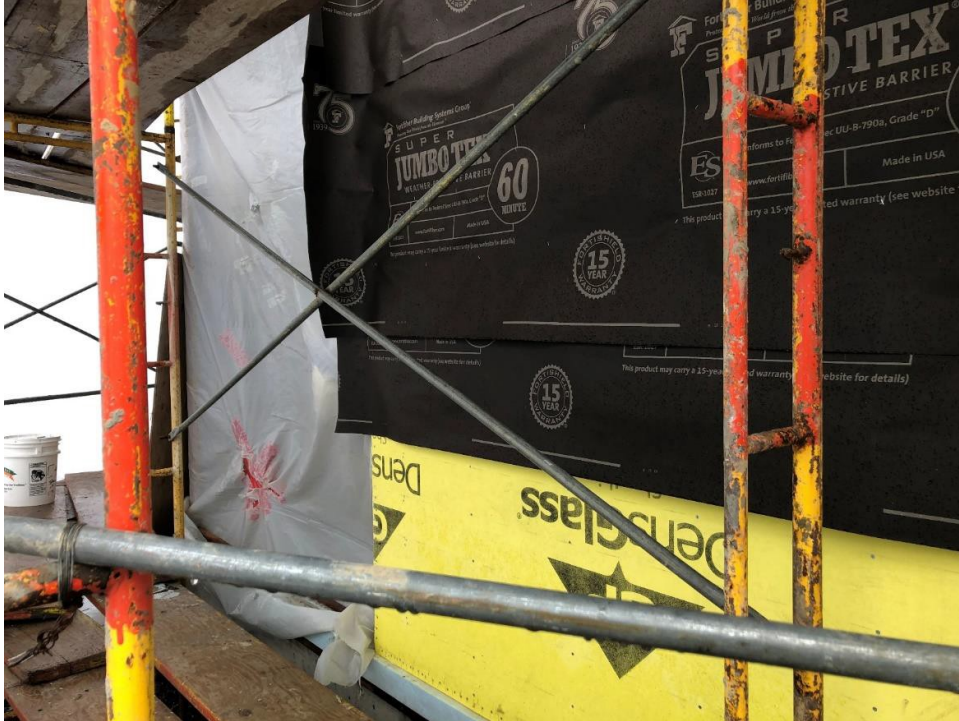
A portion of the west wall of the commons expansion exterior (Building A) showing installation of fiberglass insulation board and building paper weather barrier.
