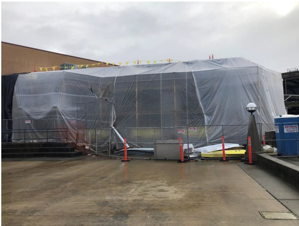
Northwest elevation of the campus additions Area A Commons (left, tented off for installation of exterior weather barrier).
