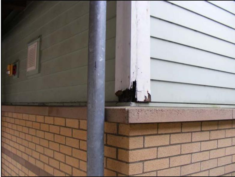
Exterior finish – wood trim is failing.
