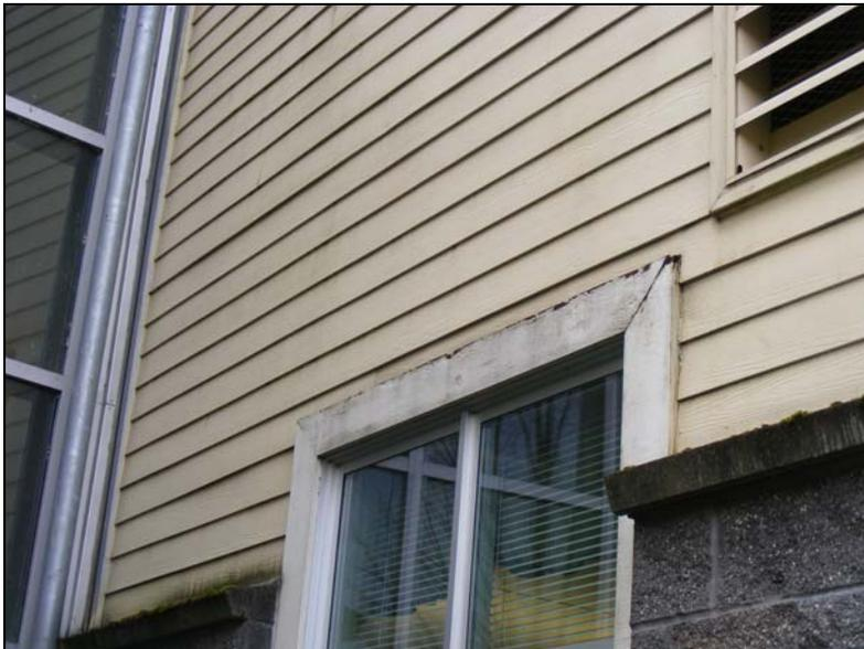
Exterior finish – wood trim is failing.
