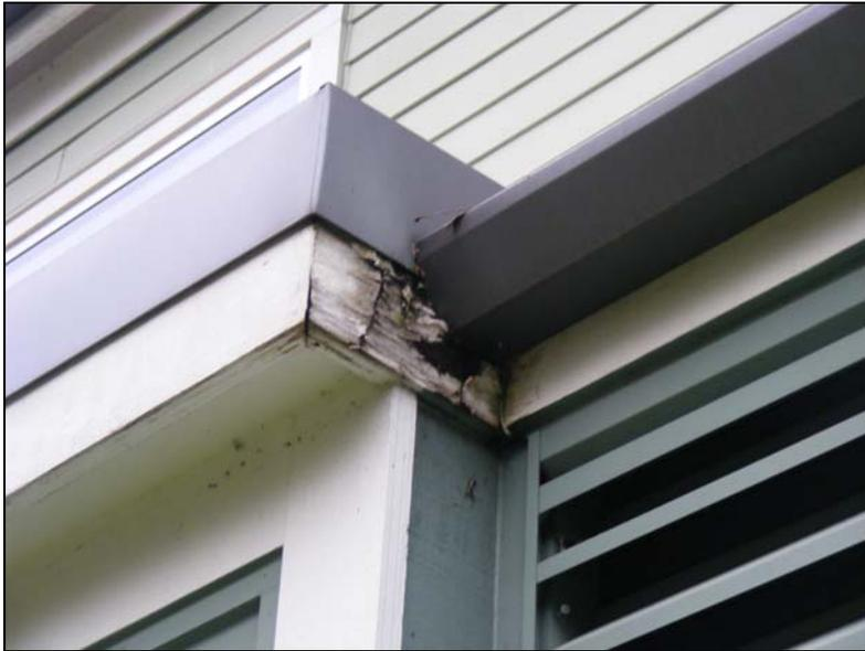
Exterior finish – wood trim is failing.
