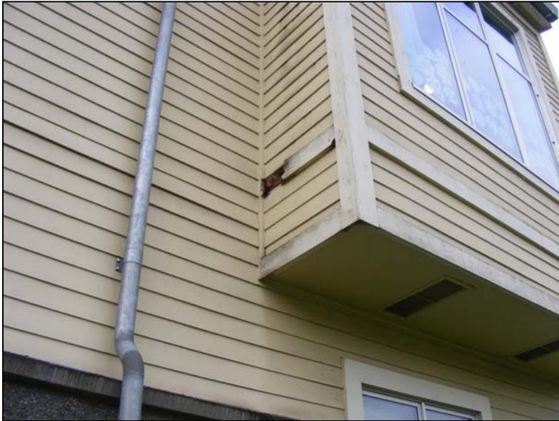
Exterior finish – wood trim is failing.
