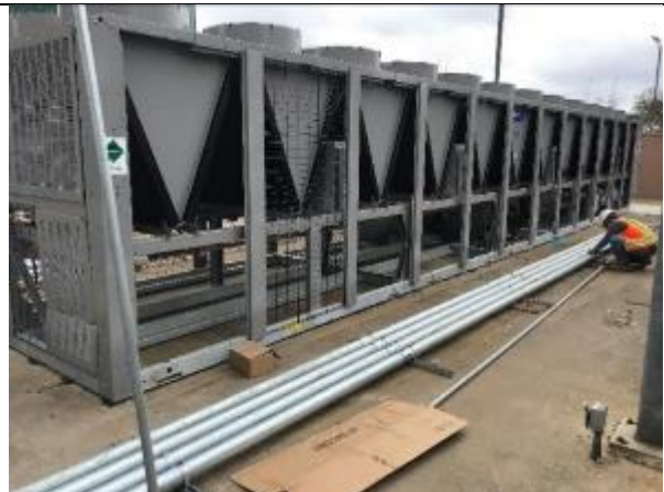
Electrical conduit is being run to the new air-cooled chillers.
