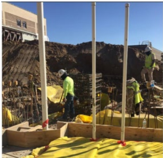
Upper seating retaining work has commenced.
