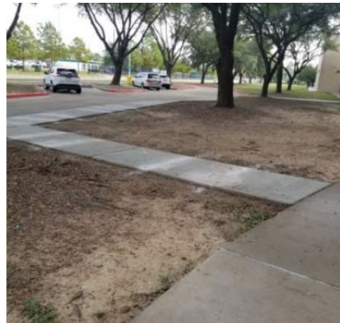
New sidewalk and storm drain relocation at entry has been completed.
