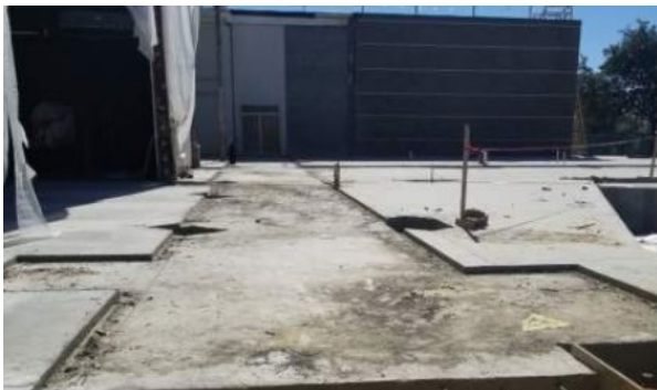
Concrete poured in Area B.2. Depression for future terrazzo.
