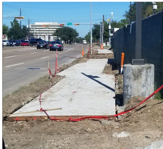
Replacement of sidewalks along Dairy Ashford have commenced.
