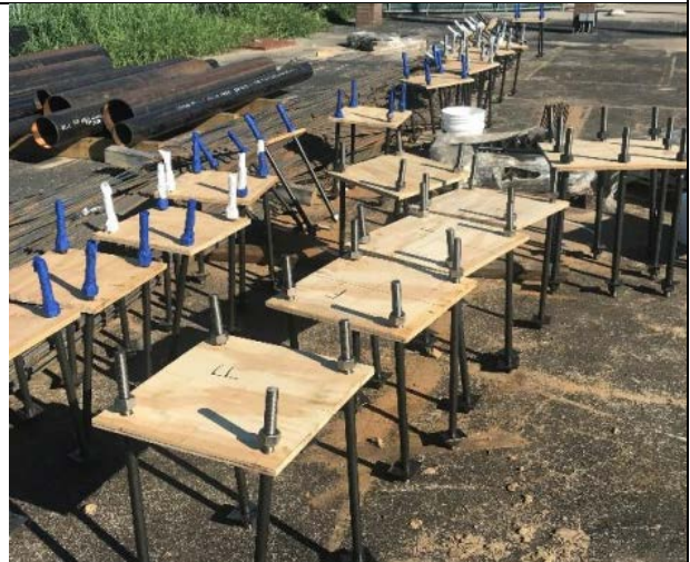
Pier reinforcing cages and pier anchor bolts are being fabricated on-site.
