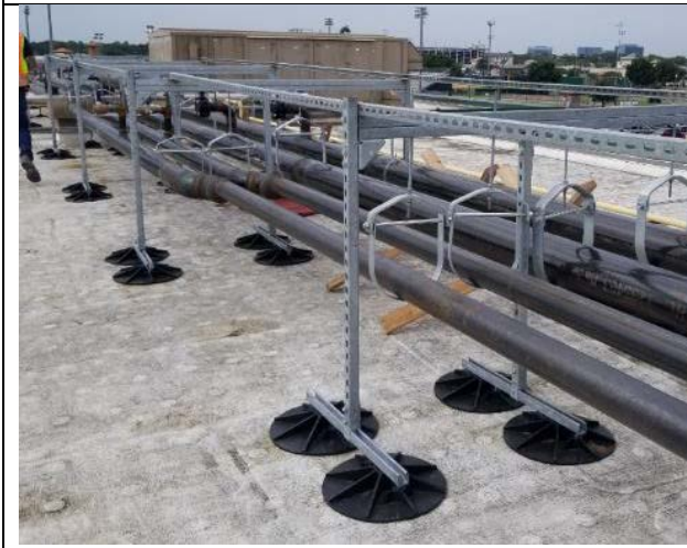
Hydronic Piping – 50% insulated
