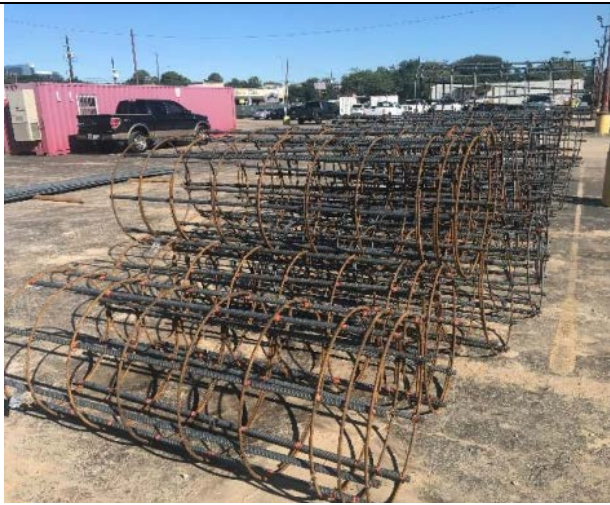
Pier reinforcing cages and pier anchor bolts are being fabricated on-site.
