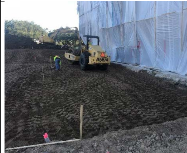
The new building pad subgrade is being compacted.
