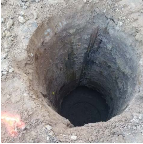
Drilling for 90+ piers of the auditorium has started.
