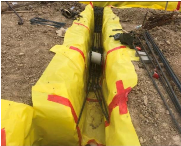
Grade beam & vapor barrier is being installed.
