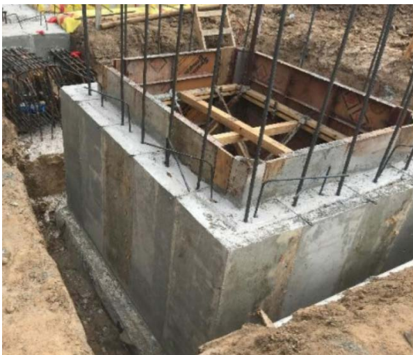
Elevator sidewalls have been poured and awaiting the waterproofing membrane application.
