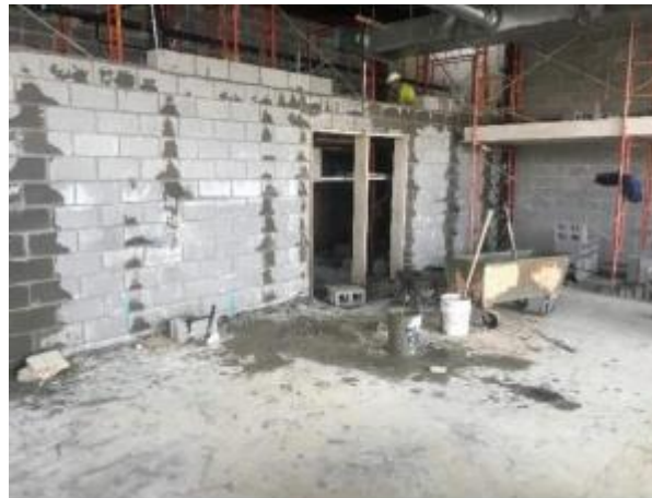
CMU block is being placed along corridor B126.
