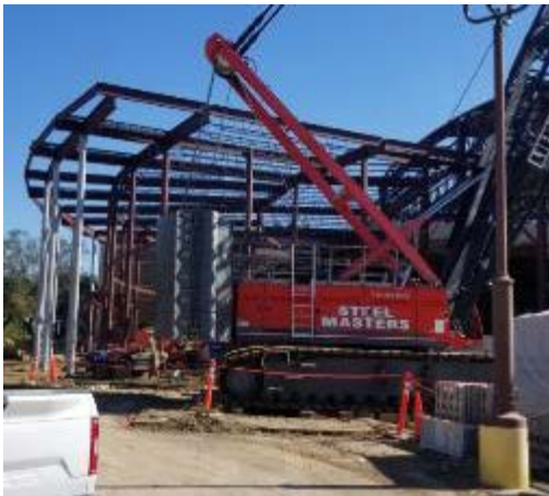
Phase 5 steel being erected.
