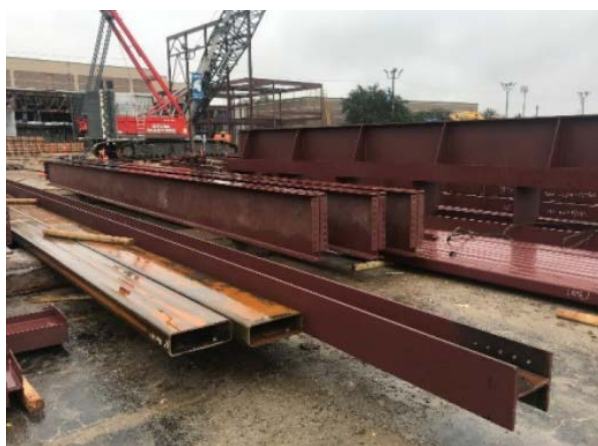
Steel beams and columns on site for Phase 2 and 3.
