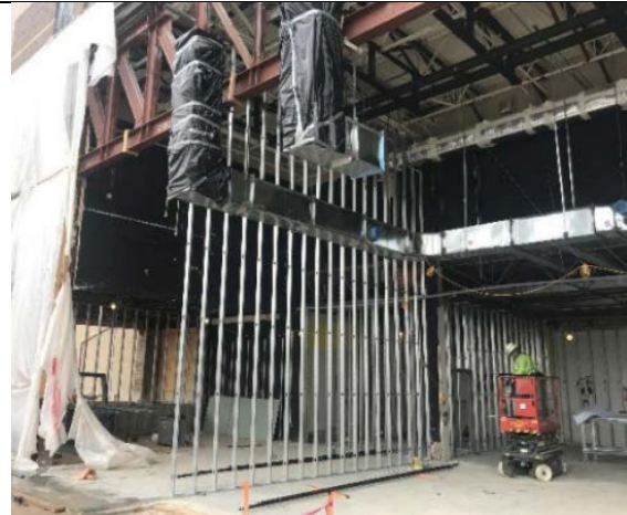
The new ductwork has been wrapped in plastic to protect against water infiltration. Metal stud work under the existing structure has started.
