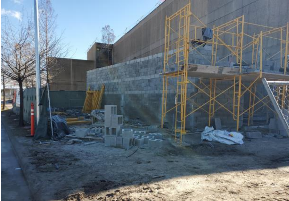
CMU block for the chiller yard currently being installed.
