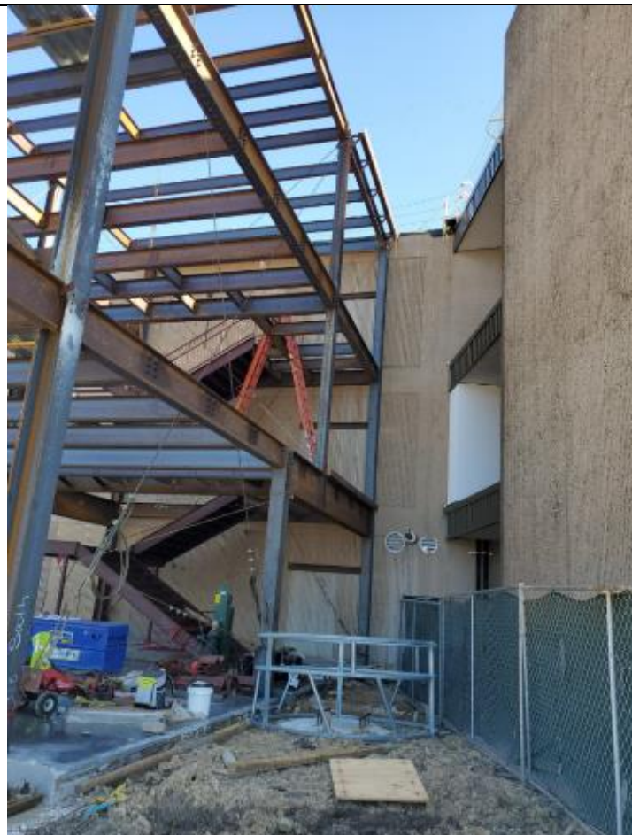
Phase 1 steel frame next to the existing North stair tower.
