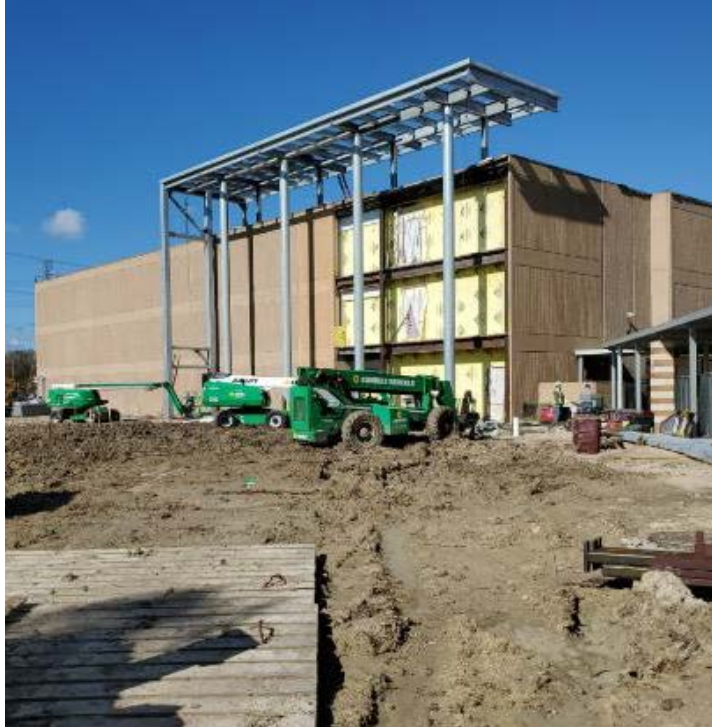
Structural frame for new main canopy has been erected.
