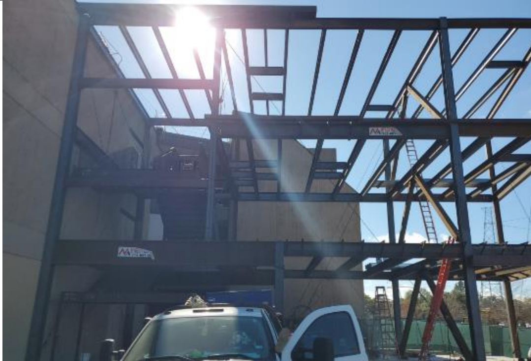
Structural steel frame for phase 1 of the addition has been constructed.
