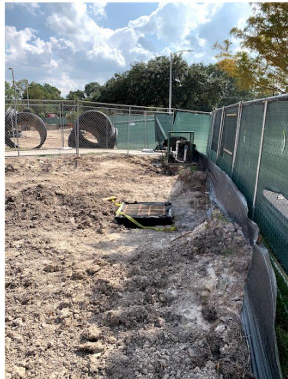
Grate inlet being installed for the underground detention
