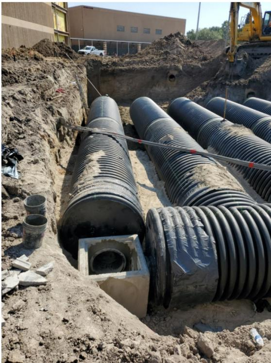
HDPE piping being installed for the underground detention
