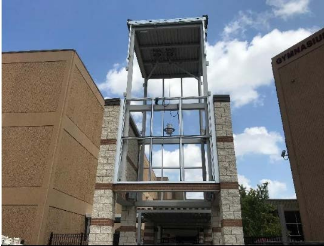
Demolition of the existing entry tower has started.
