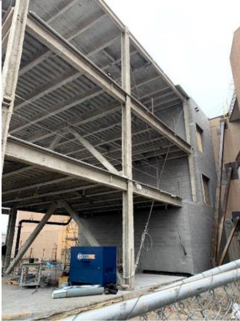
CMU block installation on-going at Phase I building addition.
