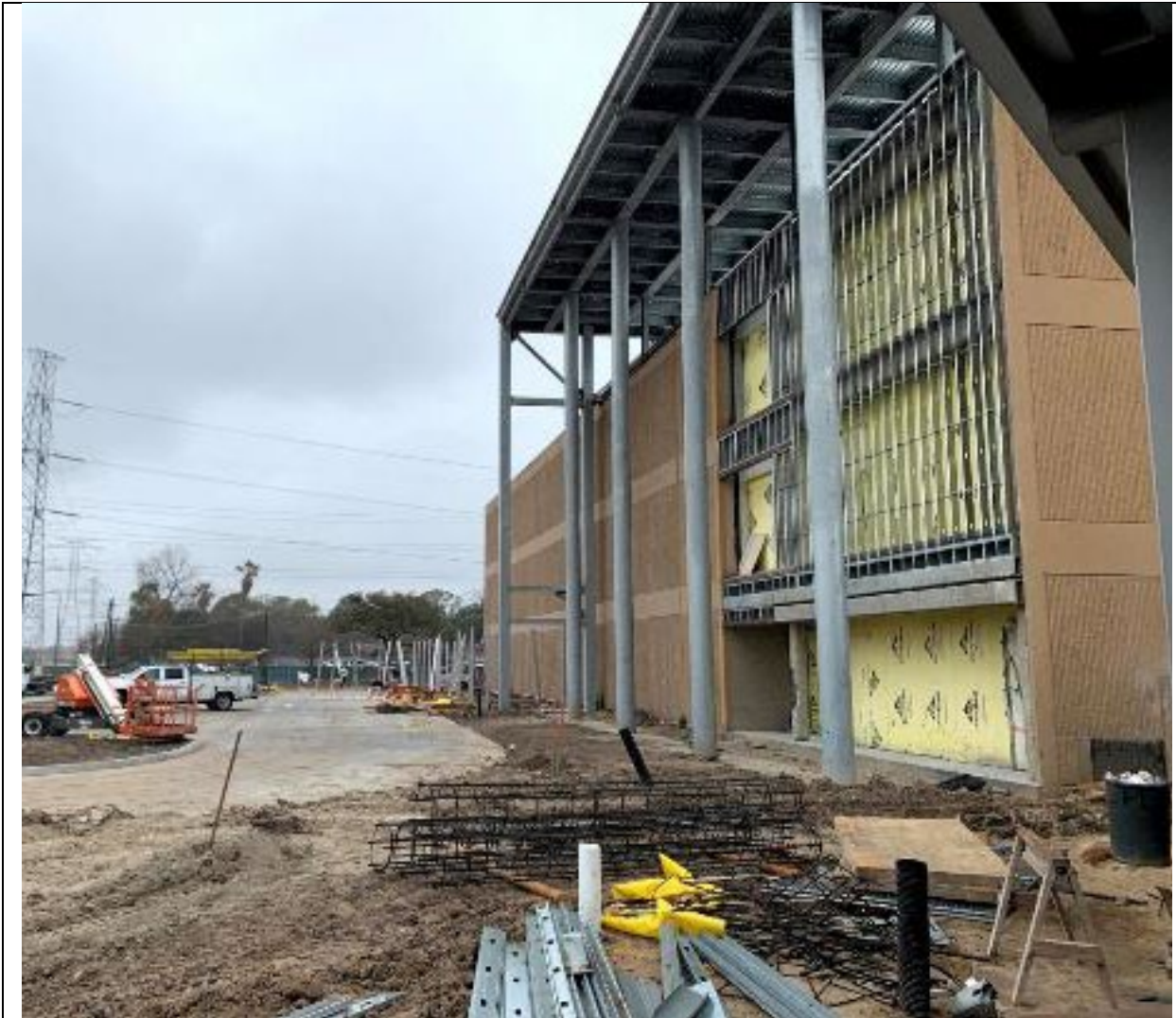
Cold rolled metal stud work at the front entry is on-going.
