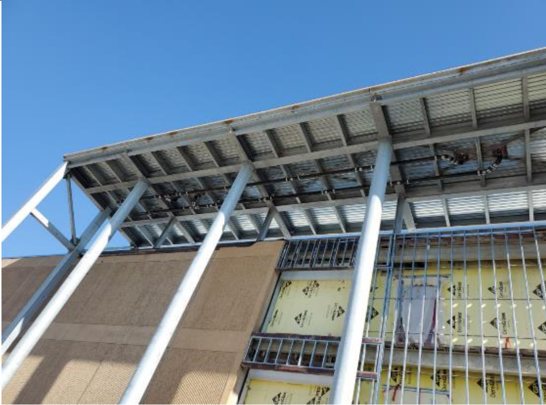
Cast iron drainage pipe being installed at the High Bay Canopy.
