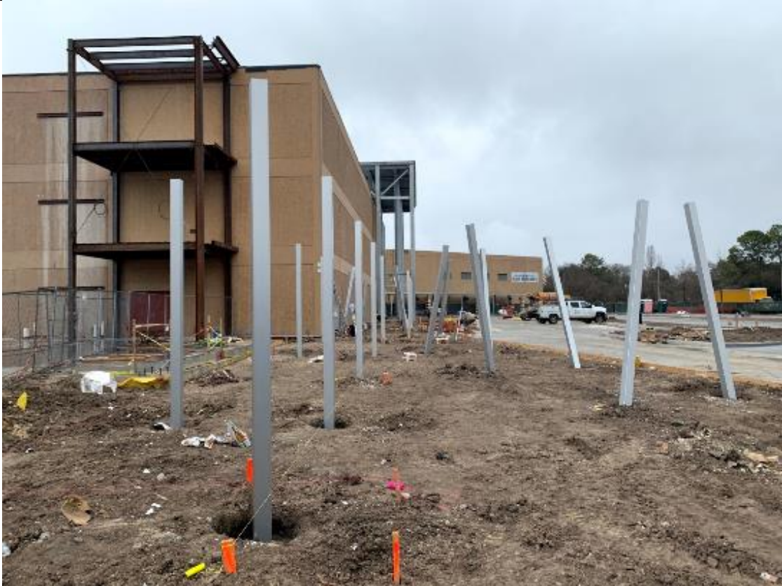
Canopy columns are being installed along the new south parking log.
