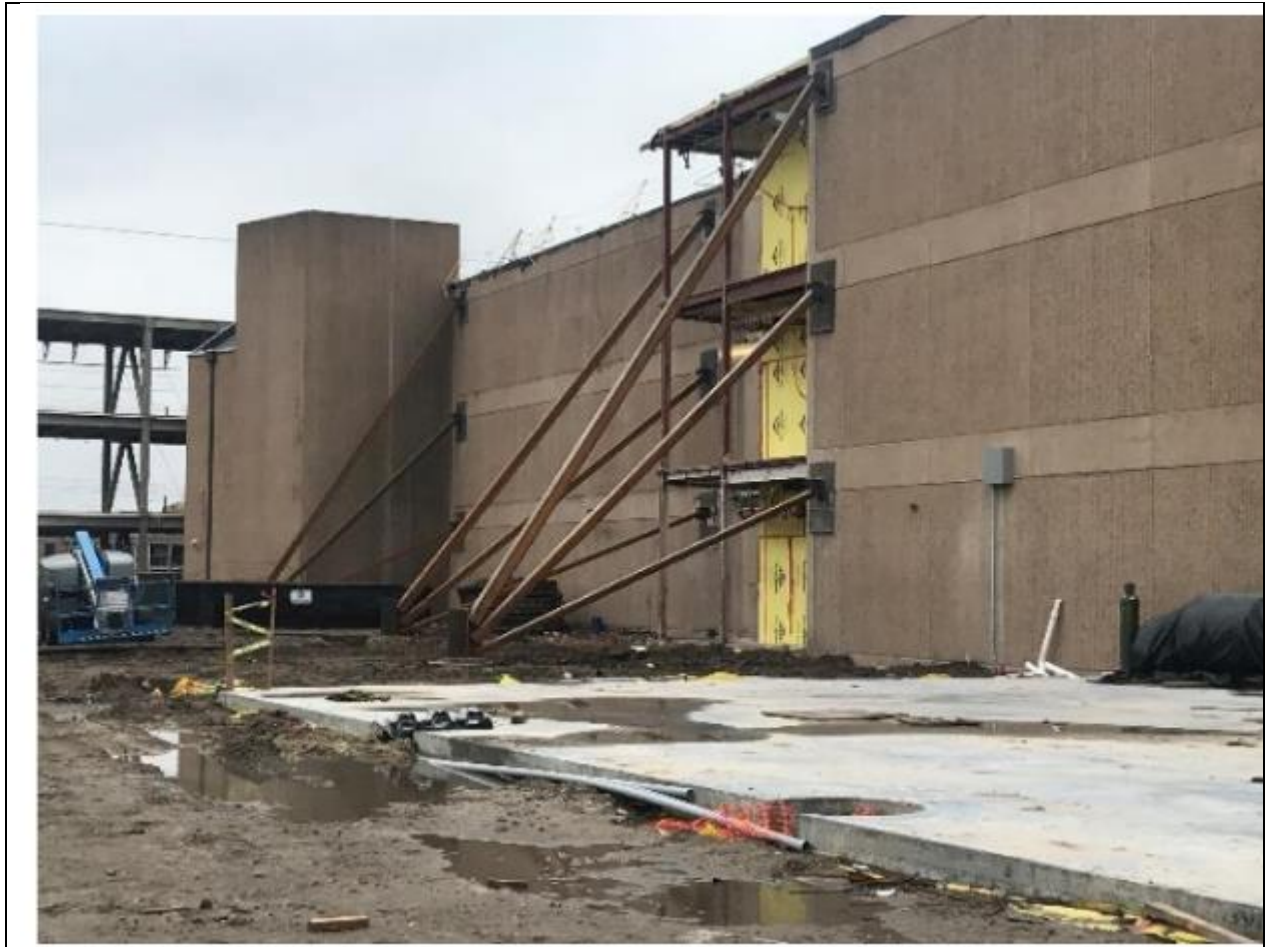
Demolition of the stair tower was completed.
