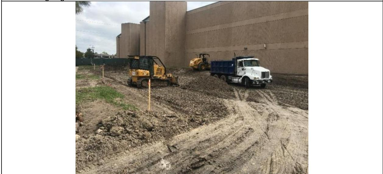
Select fill is being imported to the site and compacted in the existing detention pond basin.
