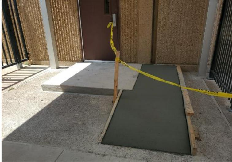
Accessible ramp has been poured at the exit door near the temporary vestibule.
