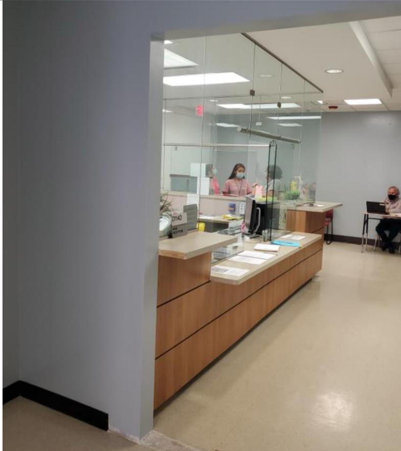
Existing door removed and opening created in the existing reception to create a temporary vestibule.
