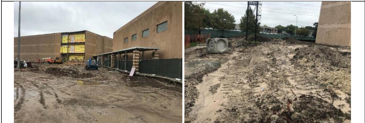
Concrete sidewalks and asphalt paving have been demolished. Underground storm sewer and manhole work is on-going
