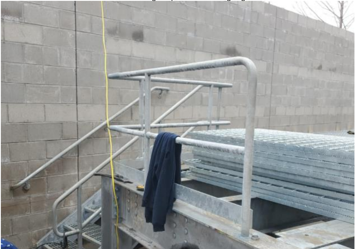
Metal stair and handrail installed at the chiller yard.
