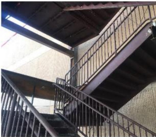
Stairway D121 stair pans have been erected, poured, and guard & handrails have been installed.
