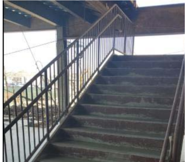
Stairway D121 stair pans have been erected, poured, and guard & handrails have been installed.
