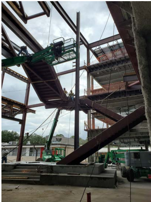
Installing atrium stair
