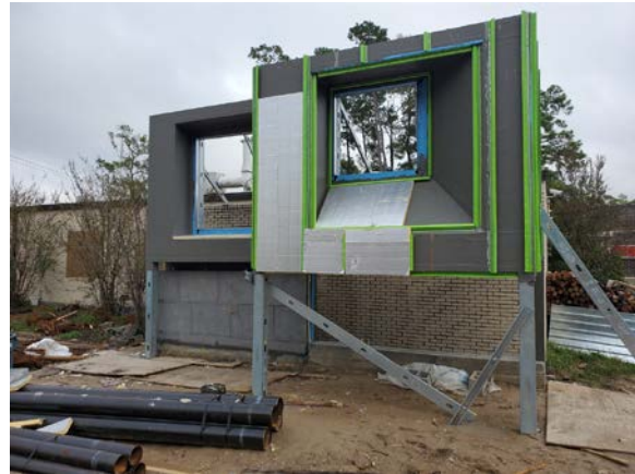
Building mockup in progress
