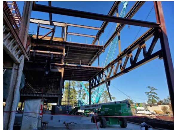
Long span truss being installed
