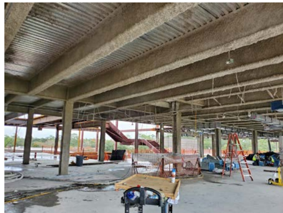
Level 3 spray fireproofing
