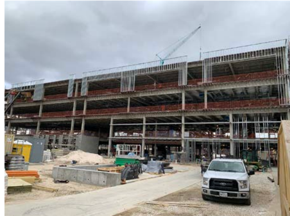
Overall west façade showing metal studs (CFMF)
