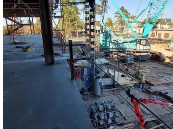
View from Level 4 at crane
