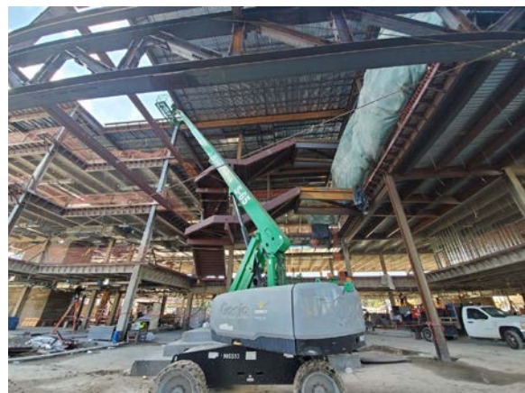
Overall steel framing from atrium
