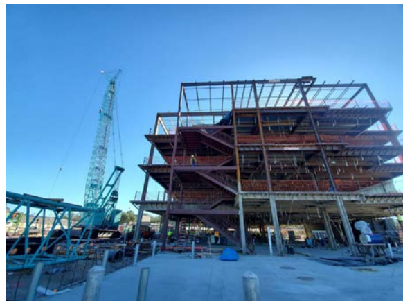
North end of the building from service yard
