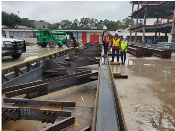
Long span truss staged on ground
