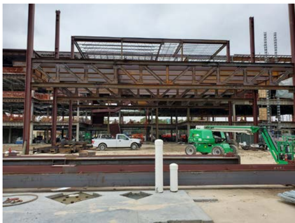
Long span trusses installed in area C
