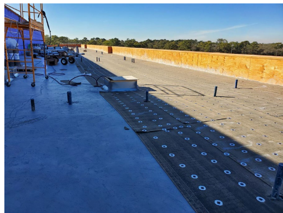
Roofing base sheet
