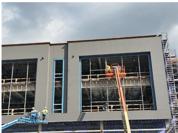
Installing window frames
