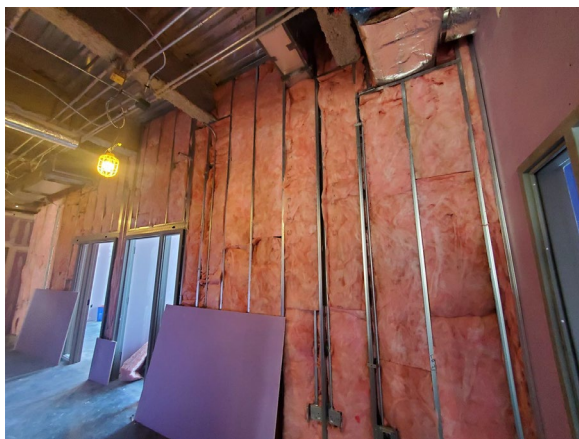
Sound insulation in walls
