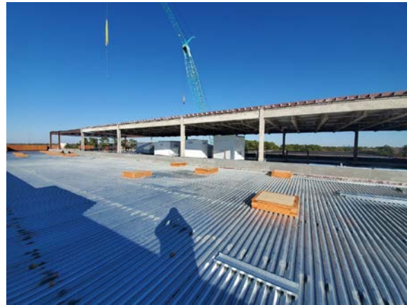
Roof over area NA
