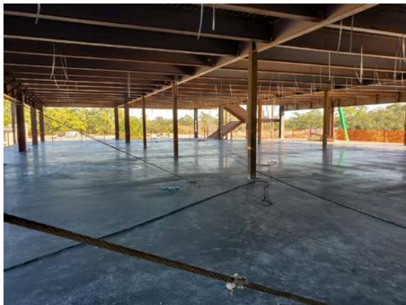
Area NC3 deck poured
