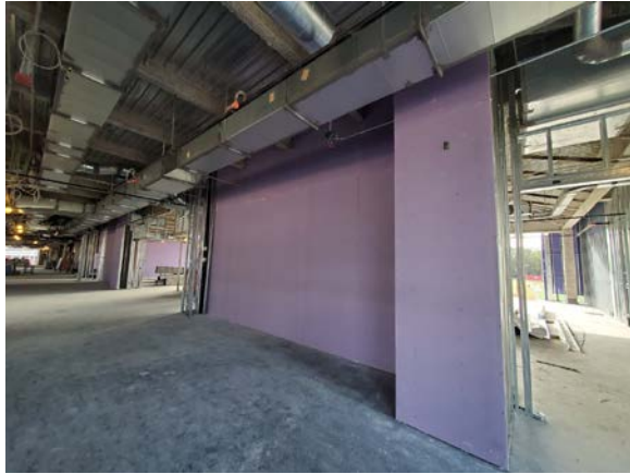
Area NA3 drywall at science labs
