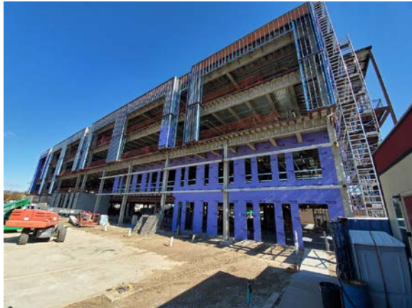
Exterior west façade
