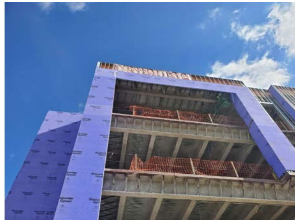
Sheathing with batt insulation at the parapets
