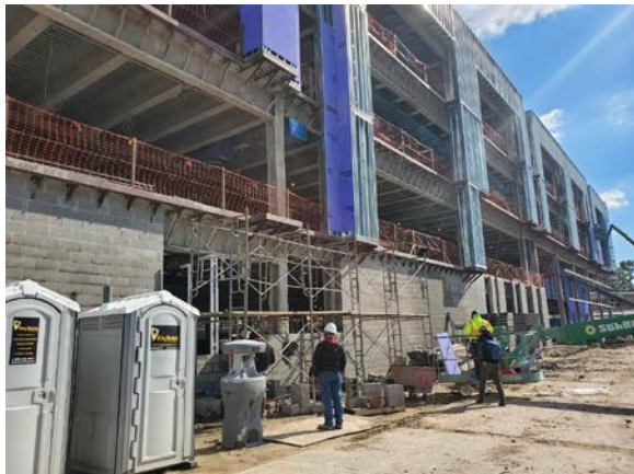
CMU work in area NA1
