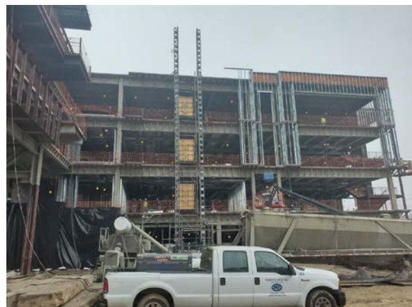
Overall Area NA (east façade)
