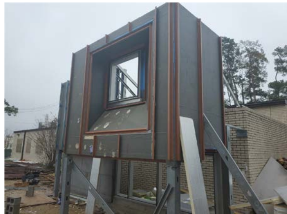
Mockup panel with replaced clips
