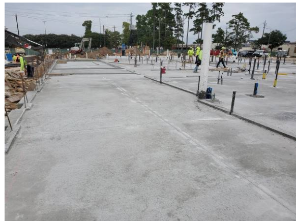
Completed slab at kitchen
