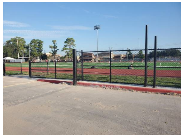
Perimeter fencing at football field
