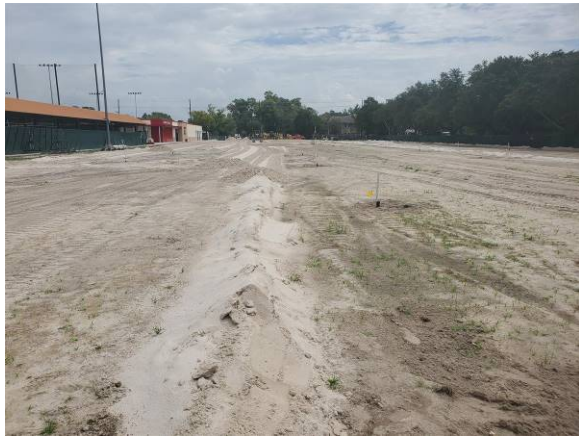
East Campus prep for sod
