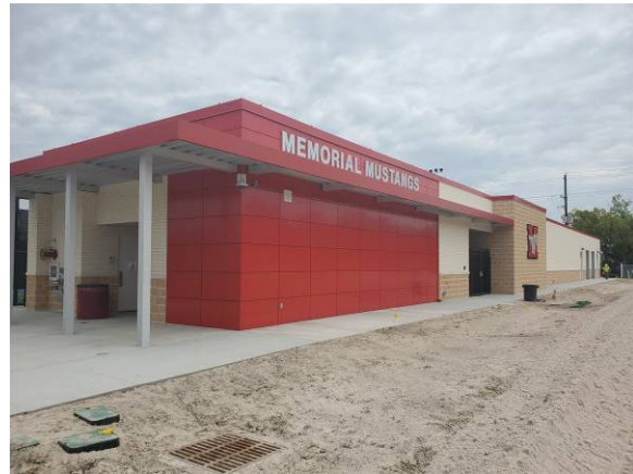
East campus prep for sod
