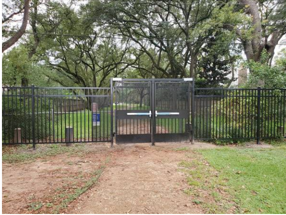
Completed secure gates at neighborhood
