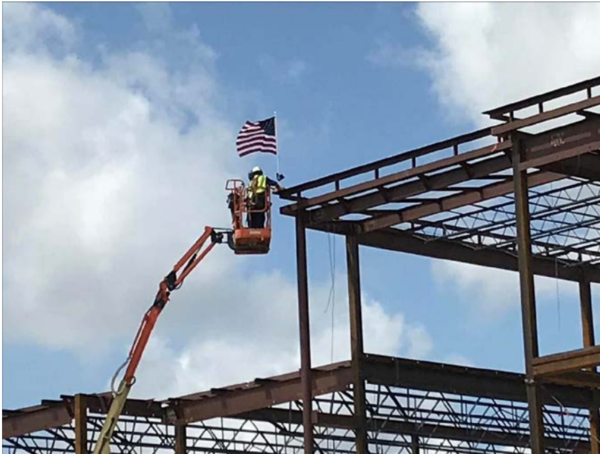
Flag is placed at building Topping Out event
