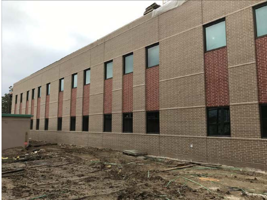
Completed brick at 2 story Admin wing
