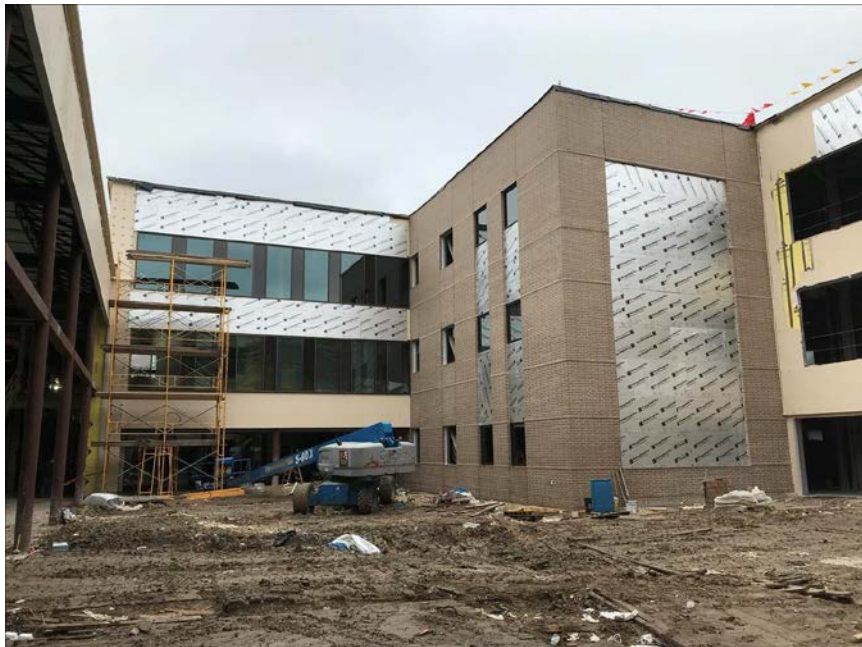
Progress at Learning Courtyard
