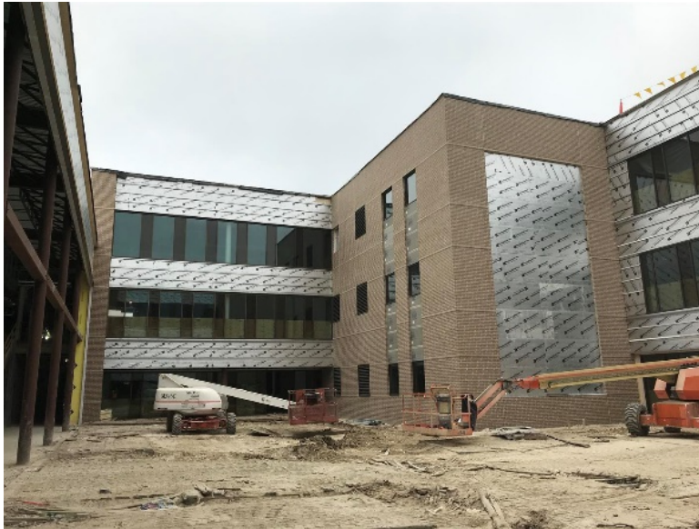
Brick, Air Barrier and Glazing at Learning Courtyard
