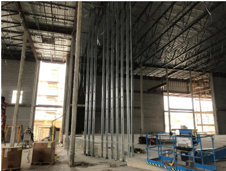
Interior Wall Framing at Auditorium underway
