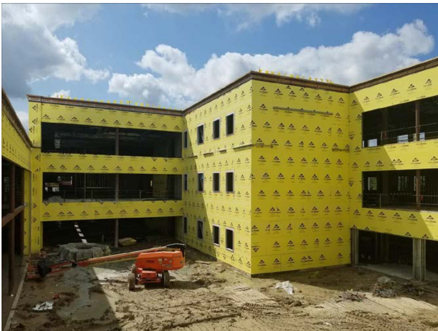
Exterior Sheathing at Learning Courtyard
