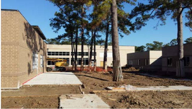
Courtyard View Progress
