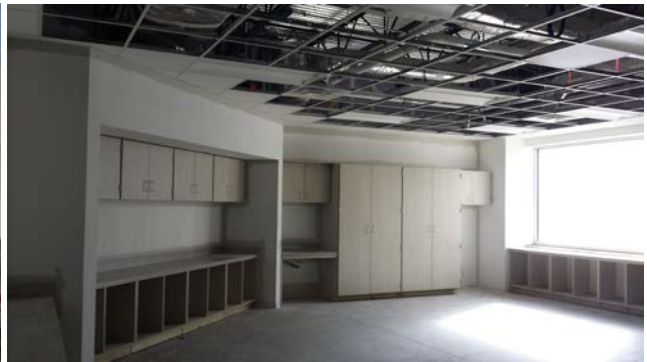
Casework Progress at Classrooms
