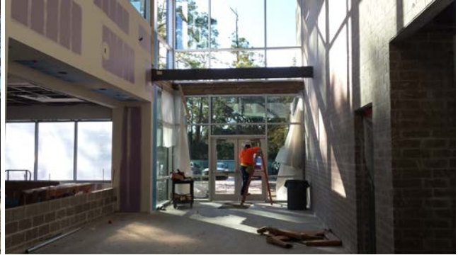
Main Entry Corridor Progress
