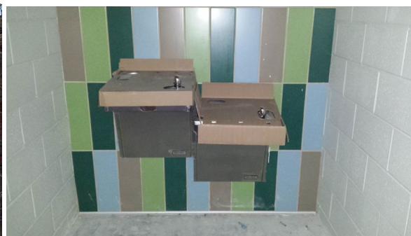
Wall Tile and Plumbing Fixture Install Progress
