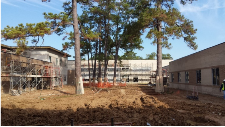
Courtyard View Progress
