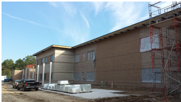
Exterior Progress At Area 'D'
