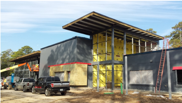
Front of School Progress
