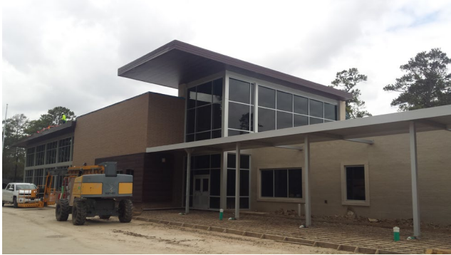
Main Entry Progress
