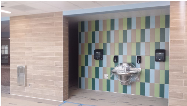
Toilet Accessories Installation Progress
