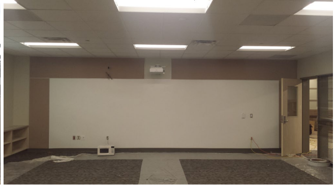
Typical Classroom- Interior Progress
