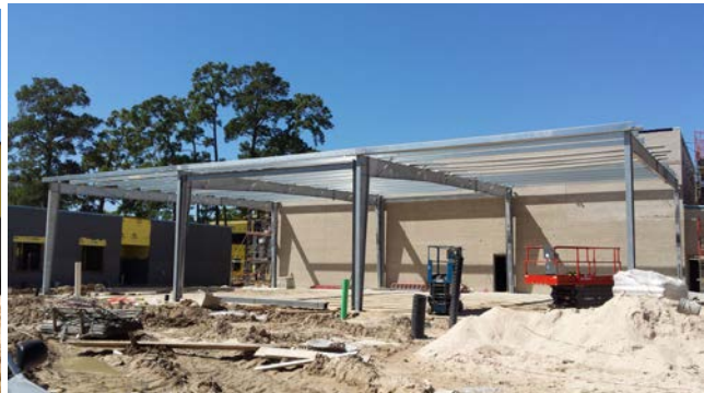
Pavilion Progress (Gym behind)
