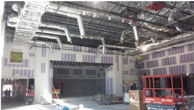
Stage/Dining Interior Progress
