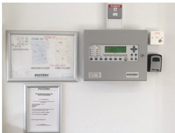
Cannon building fire alarm control panel in ground floor lobby.
