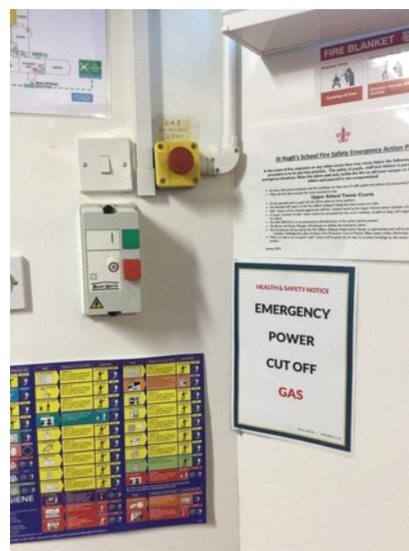
Emergency gas shut off valve in kitchen.
