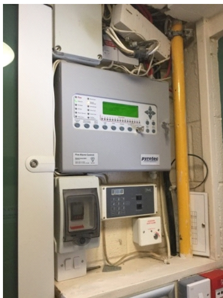
Upper school building fire alarm control panel.
