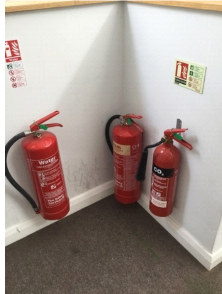
Cannon building first floor fire extinguishers missed from 2019 service schedule.
