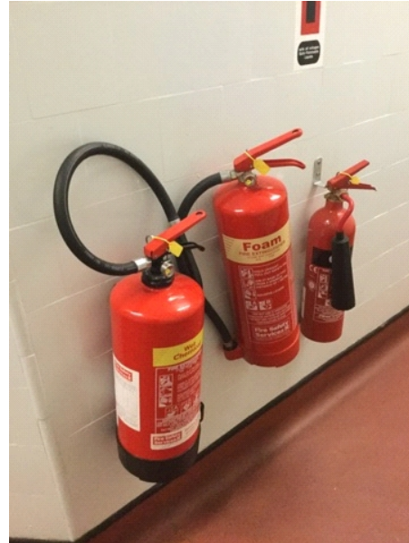
Portable fire extinguishers in kitchen corridor. Relocate wet chemical unit to kitchen area.
