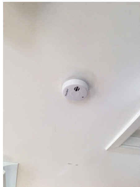
Mains powered smoke detector in French classroom (Sandbach building).
