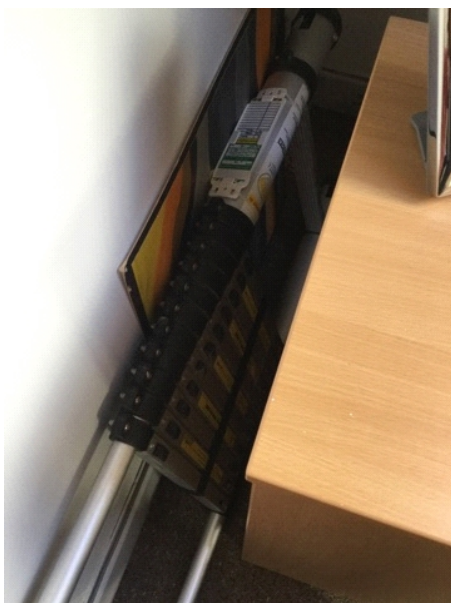
Extendable ladder for emergency exit from first floor Head of Middle school office.
