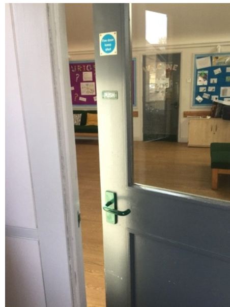
Door from ground floor Middle school to emergency escape stairwell from first floor does not close properly.
