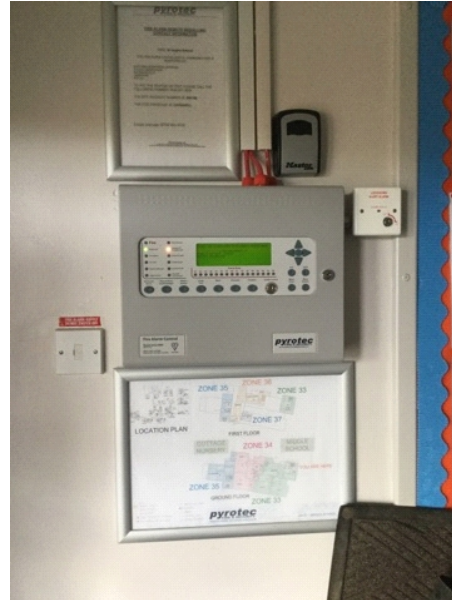
Middle school fire alarm control panel.
