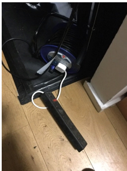
Daisy chained extension cord in drama studio next to stage.
