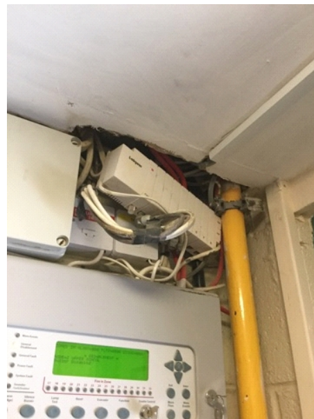
Unsupported cabling at bottom of stairs to staff room in Upper school building.
