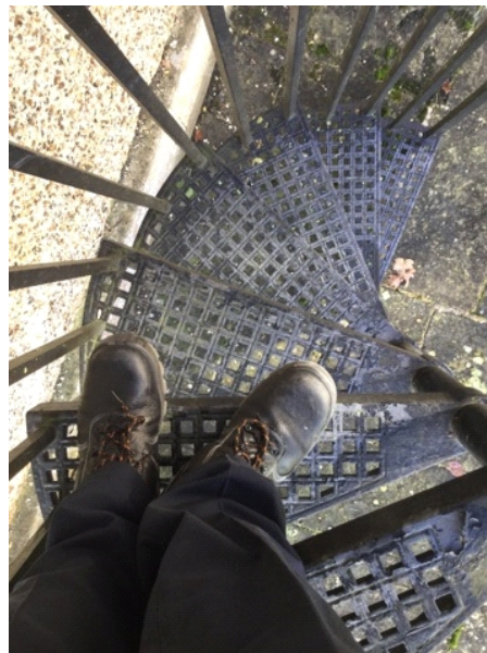
Example of small treads on external escape stairwell.
