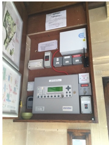
Manor House fire alarm control panel in entrance vestibule.
