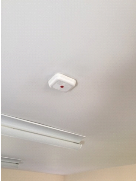
Battery powered smoke detector in General Studies classroom (Sandbach building).
