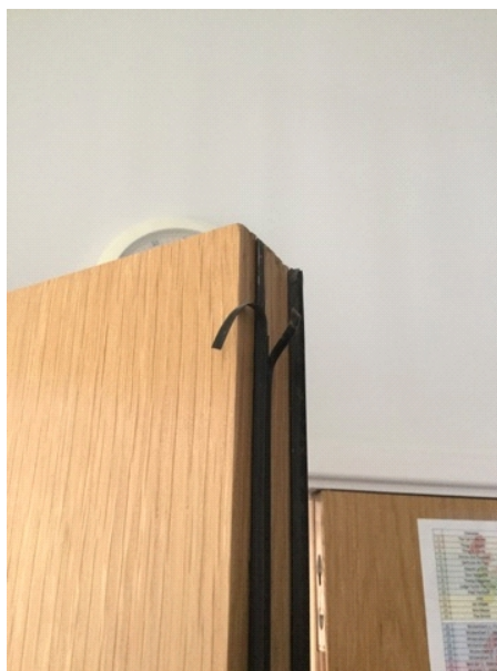
Damaged cold smoke seal on fire door to music room.
