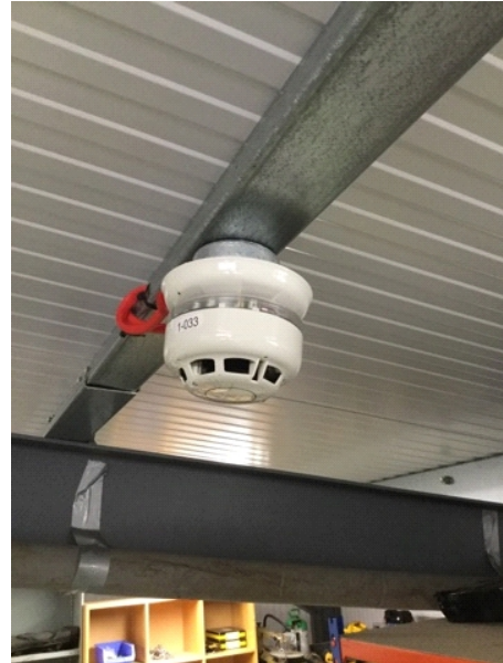
Example smoke detector and strobe warning light in grounds shed.
