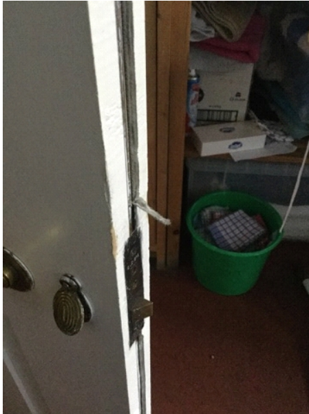
Damaged cold smoke seal on laundry room door.
