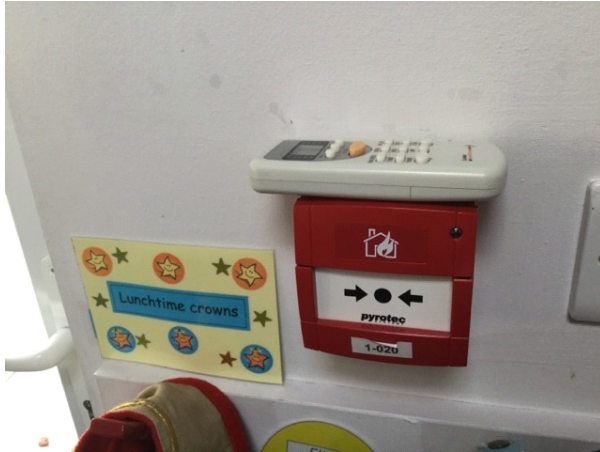
Fire alarm break glass call point next to Cottage Nursery main entrance missing protective cover to prevent false activation.
