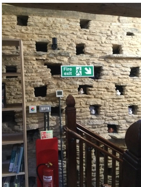
Example directional emergency escape route signage in Dovecote library.
