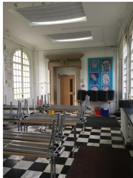
Missing directional emergency escape route signage in orangery.
