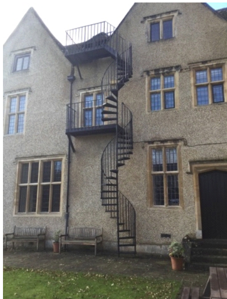
Manor House external escape stairwell. Due to steep nature, recommend only used as a last resort.
