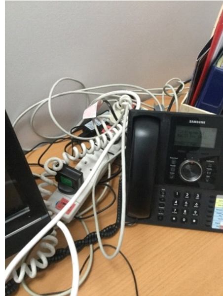
Daisy chained extension leads Head of Pre Prep office.
