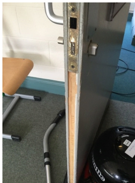
Missing cold smoke seal and intumescent strip to English 1 classroom first floor Upper school building.
