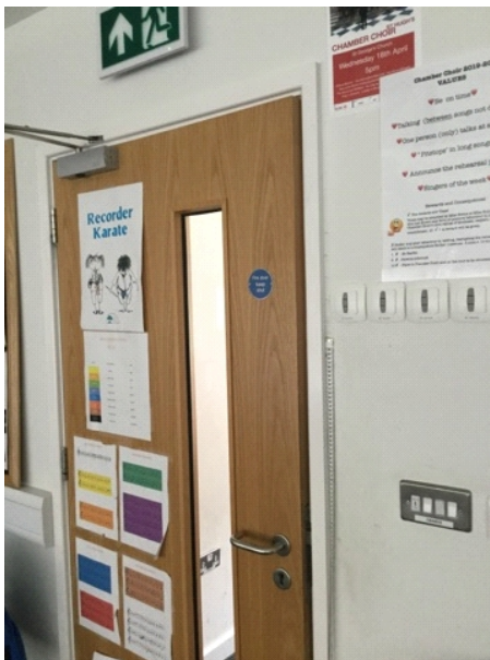
Self closer unit on door of music studio to final exit corridor needs adjusting. Door does not close properly.
