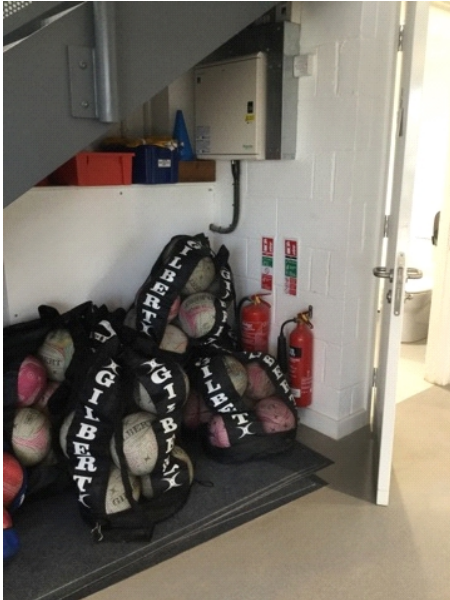
Obstructed fire extinguishers in ground floor stairwell to old side of sports hall.
