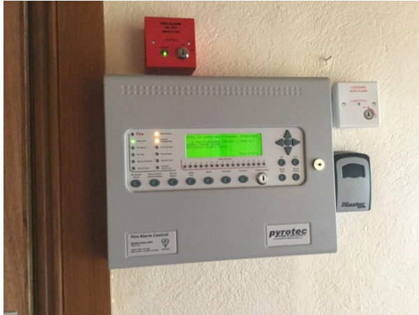
Pavilion fire alarm control panel in entrance lobby.
