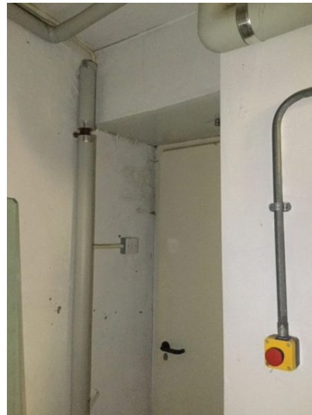
Lack of emergency lighting in Manor House boiler room.
