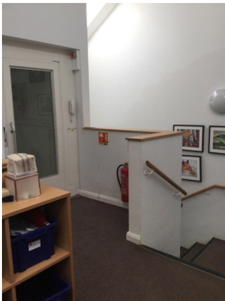
Cannon building first floor fire extinguishers not clearly identifiable.
