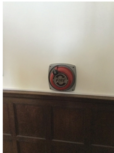
Manual fire alarm bell second floor landing main stairwell of Manor House.
