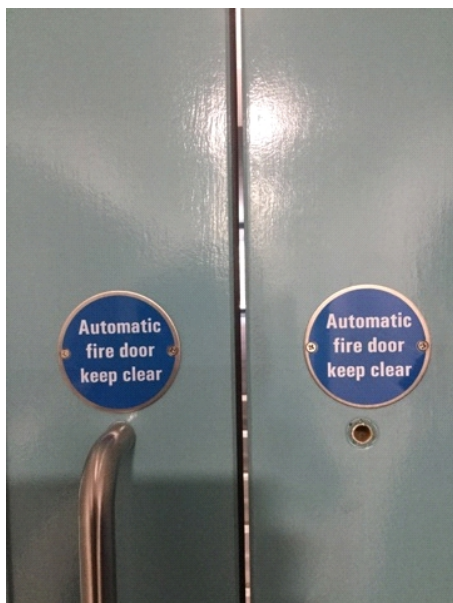
Excessive gap on doors in swimming pool corridor.
