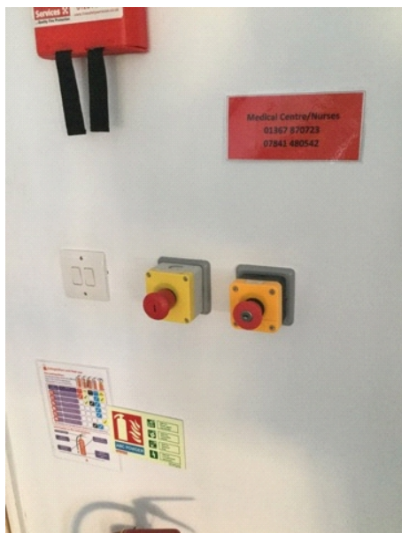
Gas and electricity emergency shut off buttons adjacent to main door to science lab 1 in Cannon building.
