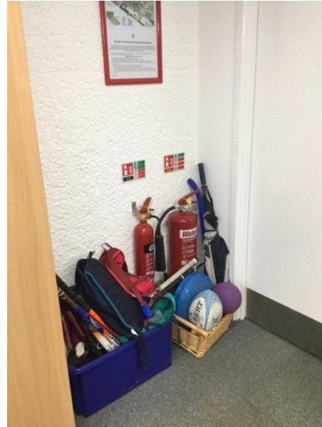
Obstructed fire extinguishers in first floor sports office.
