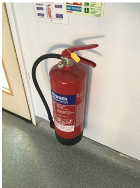
Powder extinguisher in science lab 1. Substitute for more appropriate units.
