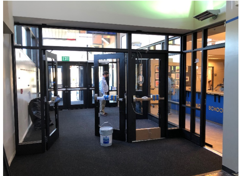
The walk off mat installation was completed today at Horizon MS.
